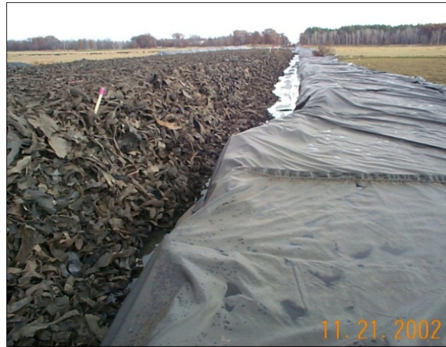
Photo courtesy of Blake Nelson, MnDOT
