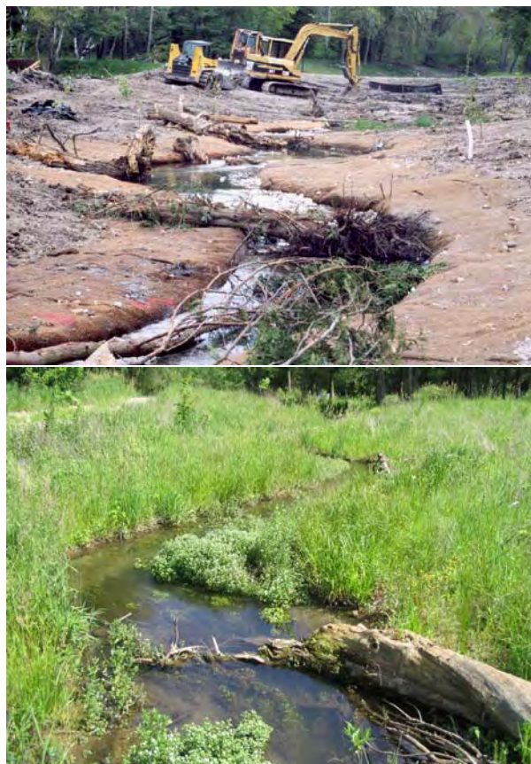
Figure 31: Stream restoration in agricultural areas can sometimes involve reconstructing a new valley form or incipient floodplain (photograph: Inter-Fluve).
