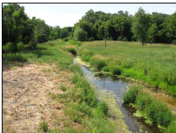
Figure 22: Reach 7, station 53300 looking upstream.
