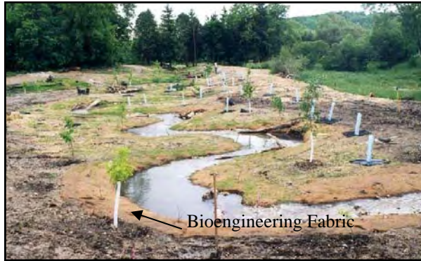
Figure 33: Grasses are beginning to grow through biodegradable bioengineering fabric along this restored stream (photograph: Inter-Fluve).
