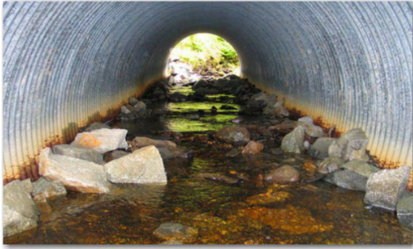
Figure 32: Bottomless arch that is partially buried for better habitat and fish passage conditions.
