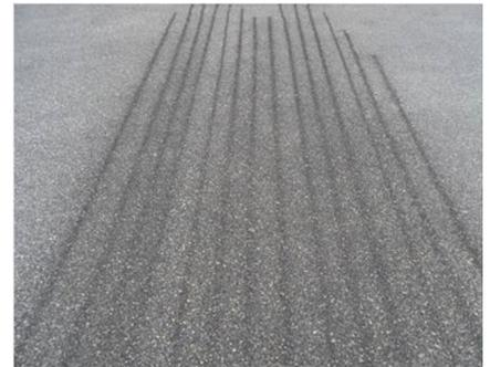
Figure 20: Wheel path anti-icing
