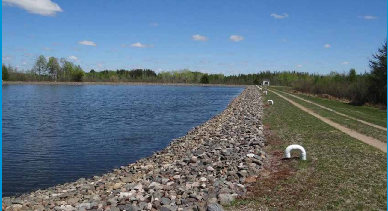
McGregor Wastewater Treatment Plant
