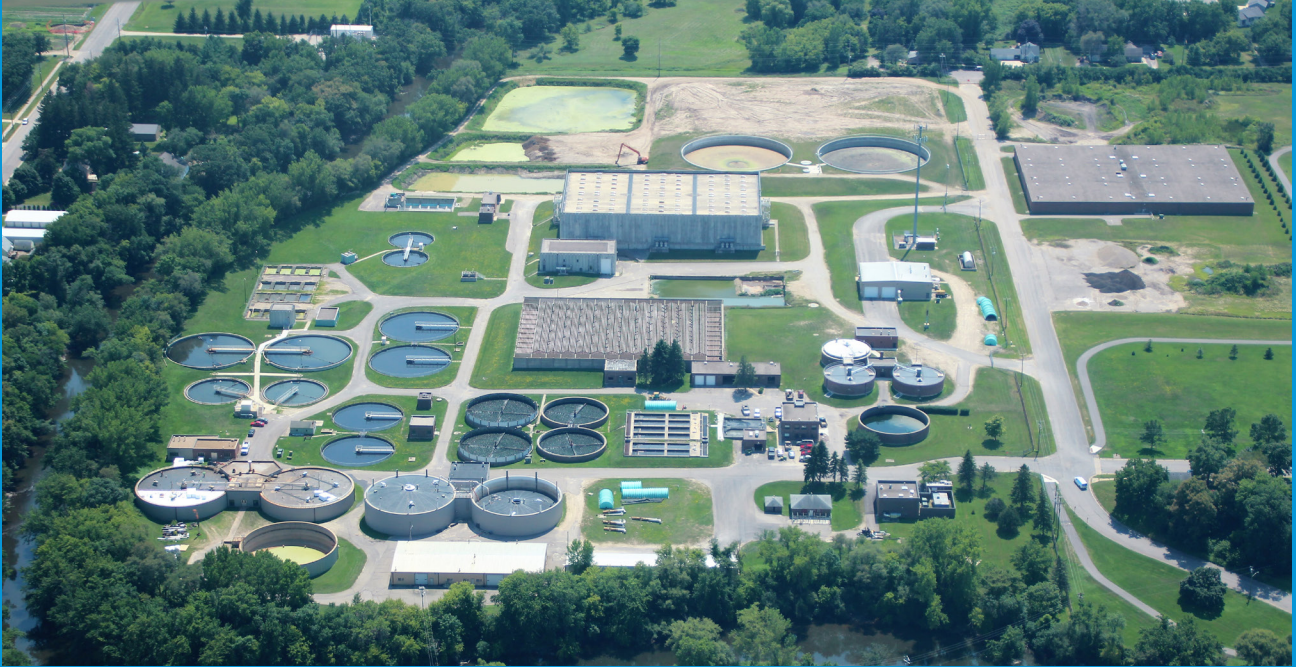
Austin Wastewater Treatment Plant
