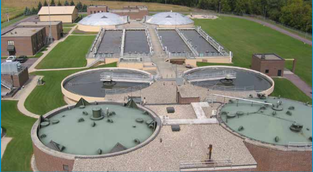
Owatonna Wastewater Treatment Plant
