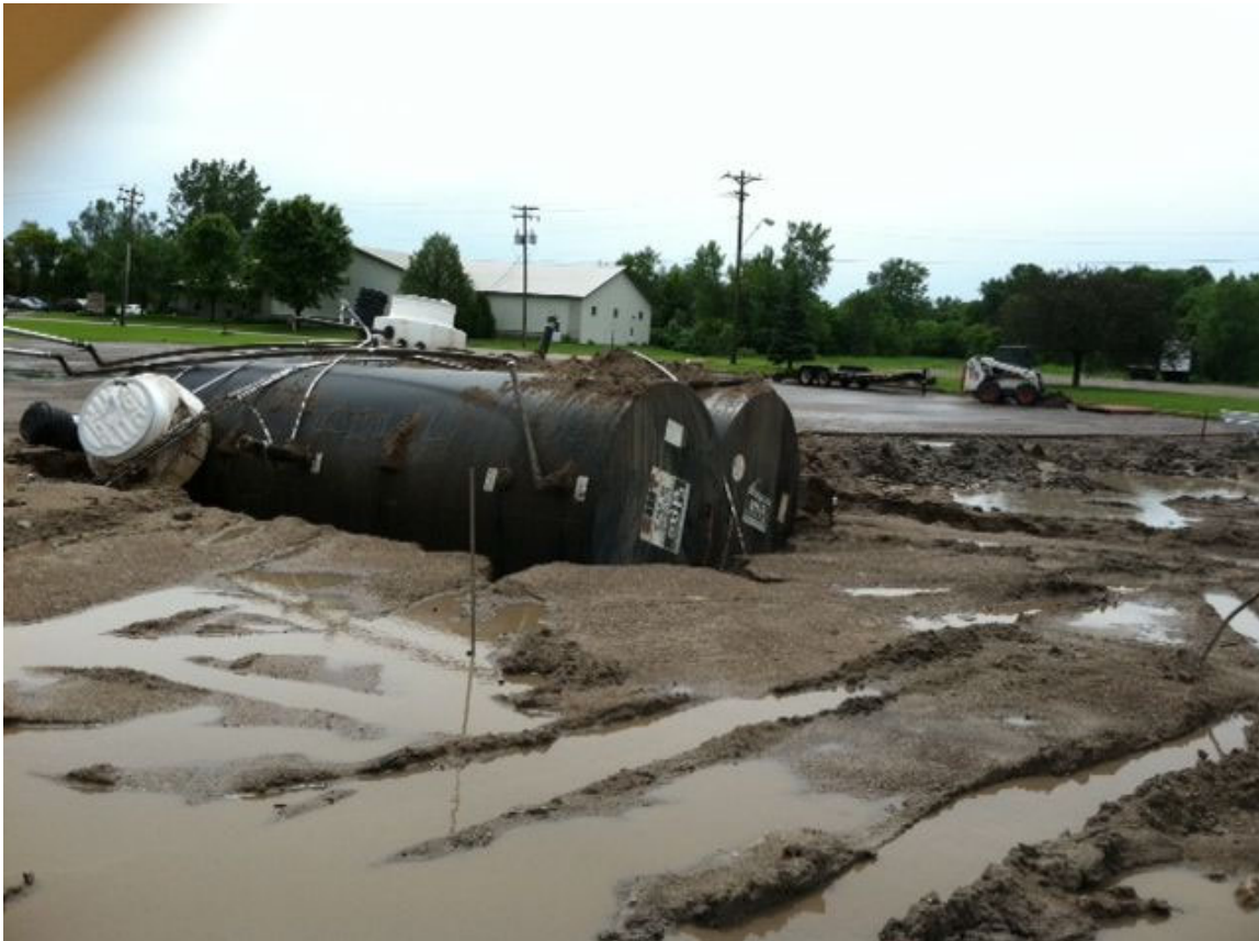
Photo: Underground petroleum storage tanks exposed from flooding in Albertville, MN (Wright County), June 19, 2014. Photo courtesy of Jake Mueller.
