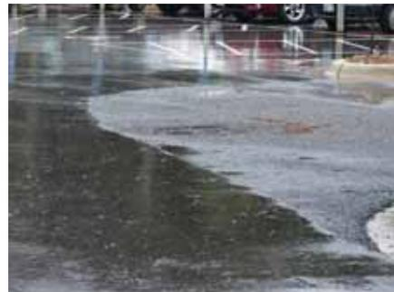
Intersection of impervious asphalt (left) and pervious asphalt (right)
