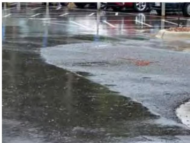
The intersection of impervious (left) and pervious (right) asphalt shows the efficient infiltration ability of using pervious pavements.
