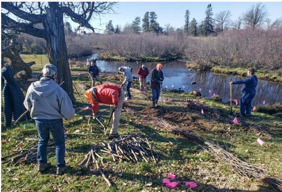
Hubbard SWCD staff and Trout Unlimited volunteers installing a stabilization planting along the Kabekona River. This area was high traffic for Cattle and had minimal vegetation. A mix of wetland shrubs and seeds mixes were planted.
