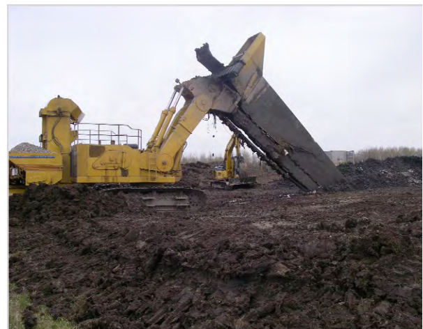
Trenching for Leachate Drain at Koochiching County Landfill
