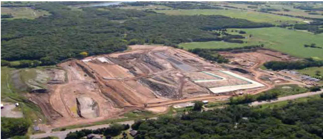
Aerial photo of construction at the Washington County Landfill
