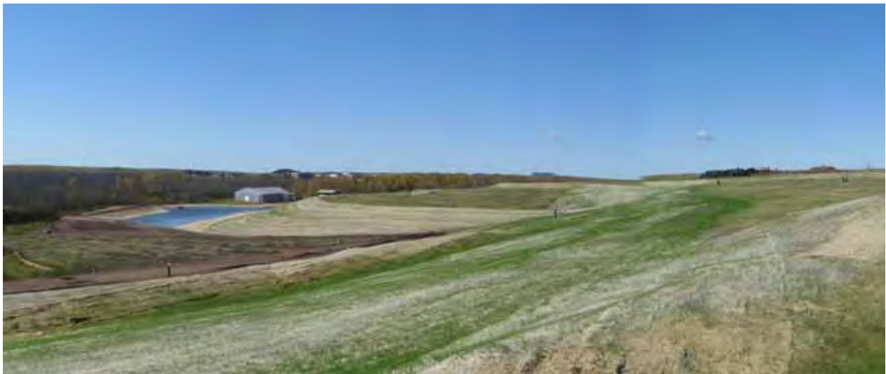
Cover construction at the WLSSD Landfill, St. Louis County
