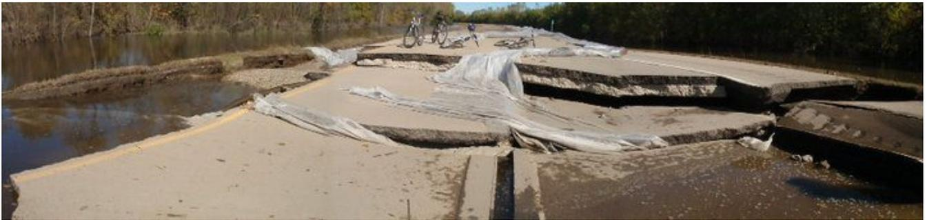
*Flash flooding in September 2010 caused Highway 169 to break apart north of St. Peter.*
