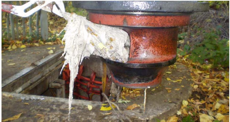
Clearing a wipes clog from a sewer-system pump in Minnetonka.
