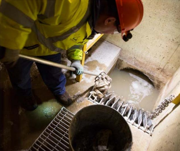
Wipes must be manually raked off a bar grate every day at a lift station in Eagan.
