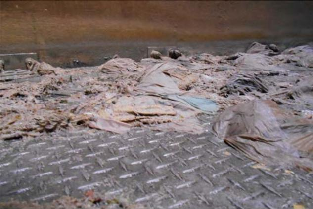
Wipes on the "trash rack" in the Rochester wastewater treatment plant. The trash rack is an early screening of material coming into the plant.
