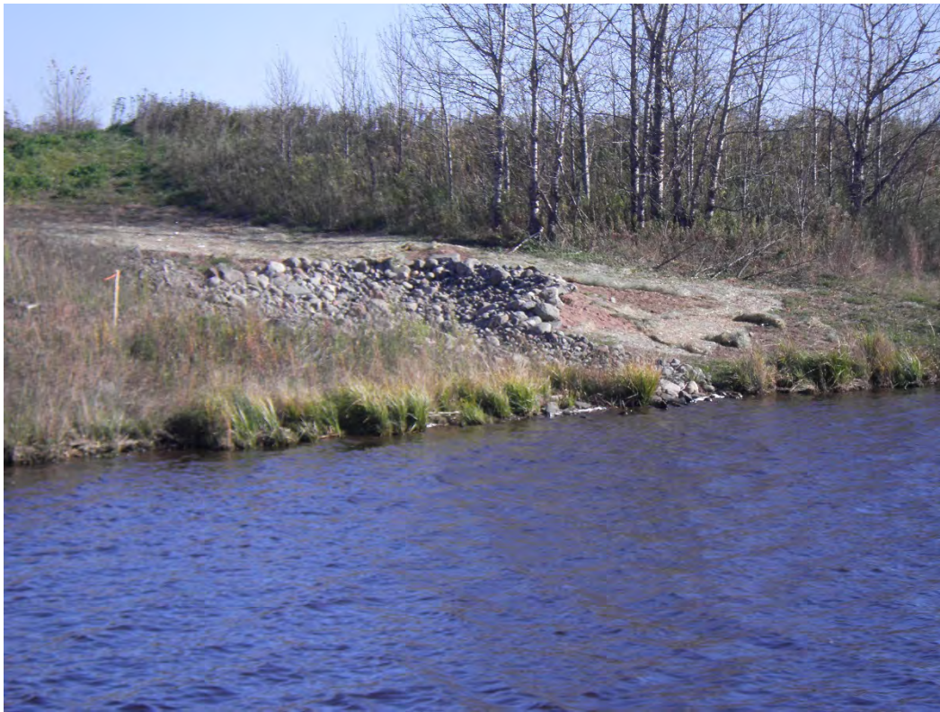
North end of CAD, erosion repair
