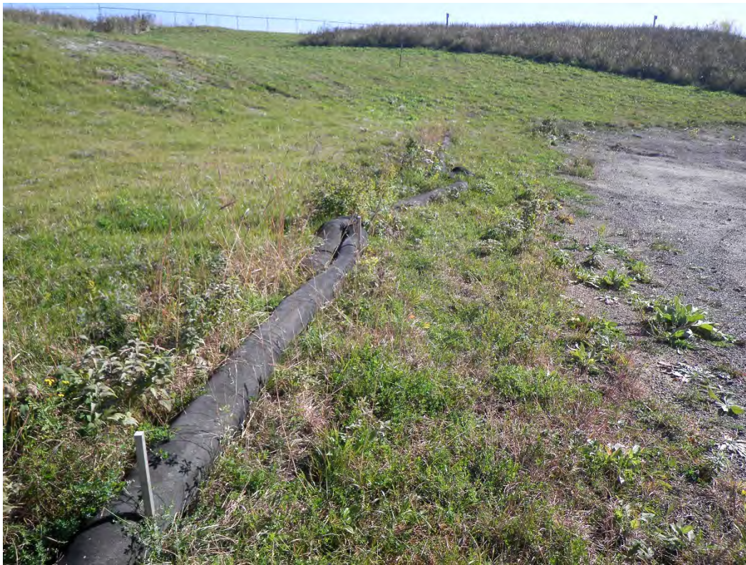
Stryker Bay hillside erosion repairs, view east
