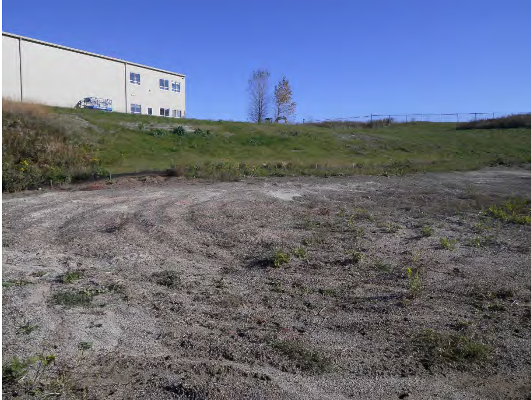
Stryker Bay hillside erosion repairs, view northeast
