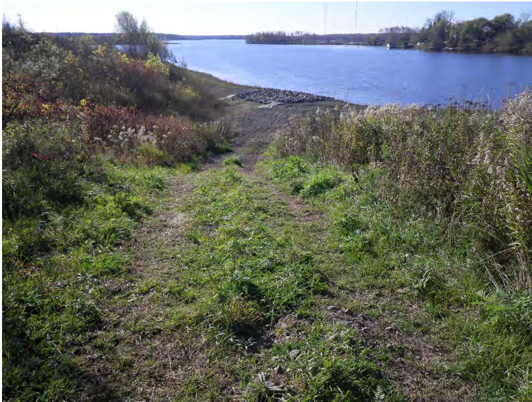
Stryker Bay, north end cap repairs
