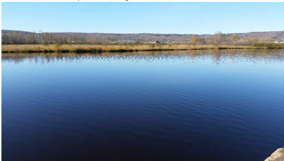
Location 24, East side of Slip 7, central, along the dock wall, 330 0
