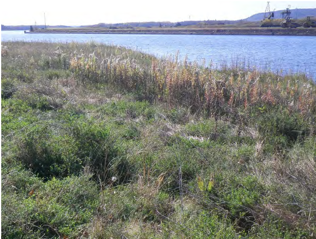
View of CAD dock wall, view southwest
