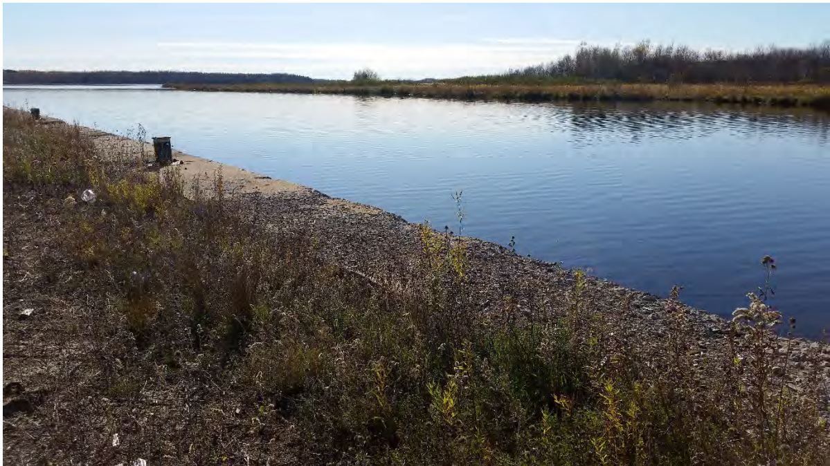
Location 23, East side of Slip 7, central, along the dock wall, 215 0
