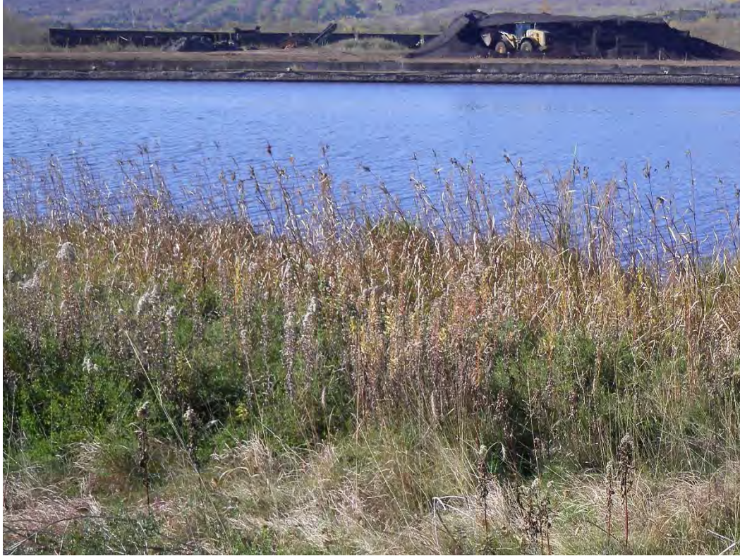
View of CAD dock wall, view west
