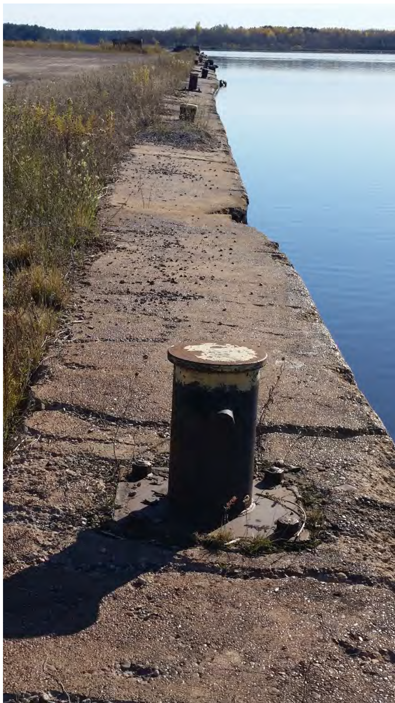
Slip 7 dock wall, view south
