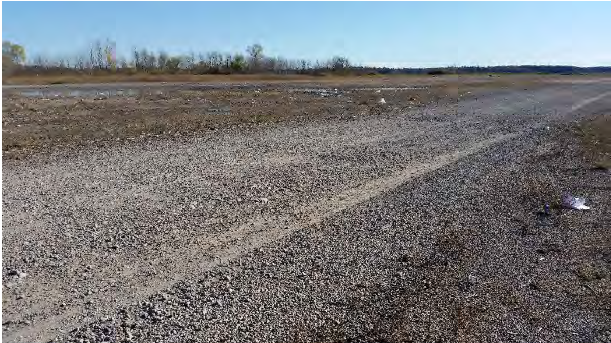
Location 23, East side of Slip 7, central, along the dock wall, 145 0
