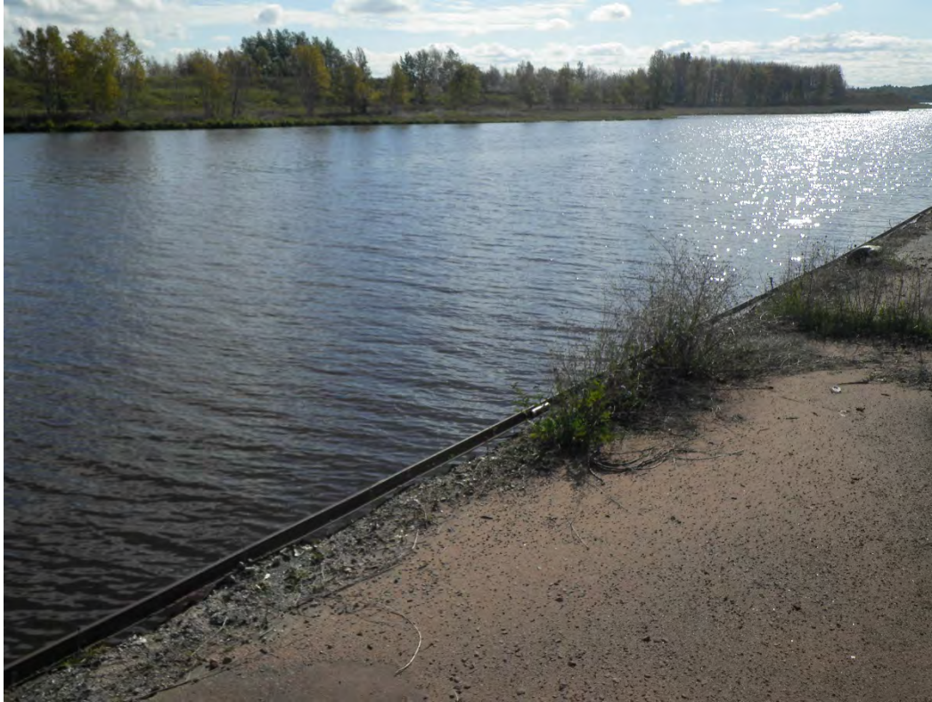
Location 9, Central dock wall along Slip 6/CAD, 145°
