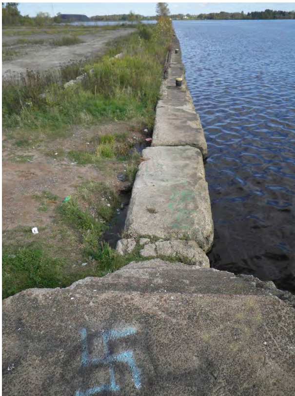
Slip 7 dock wall, view east from SW corner
