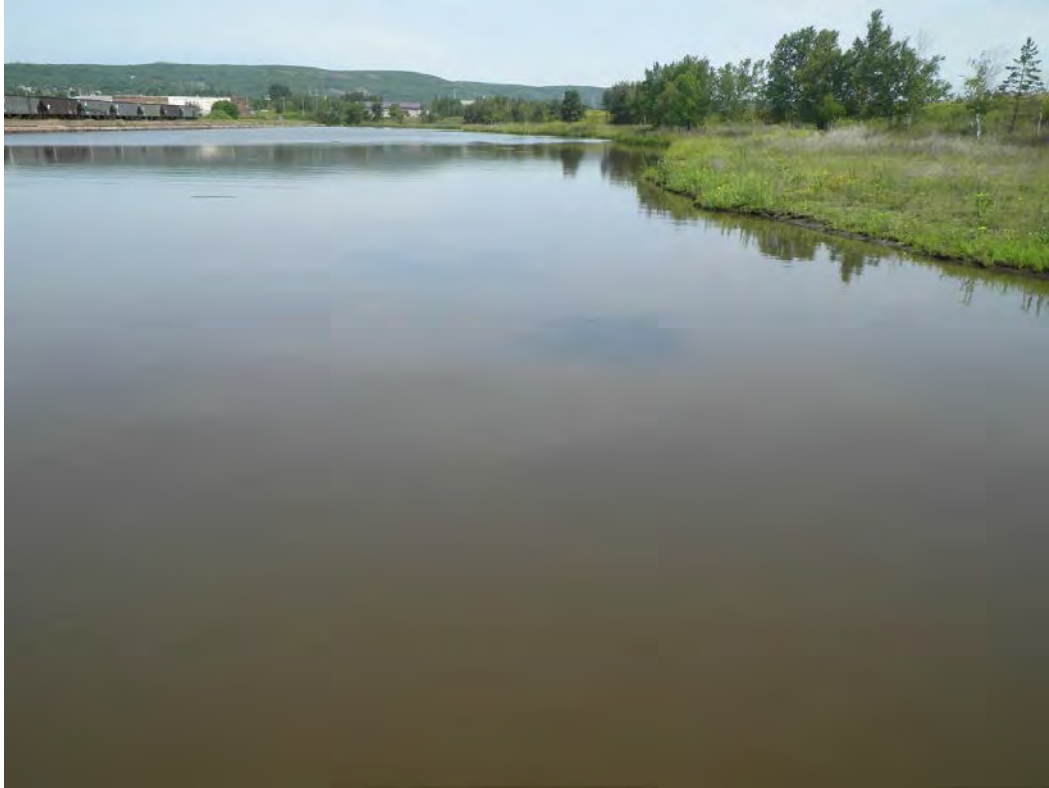
Slip 6, view north
