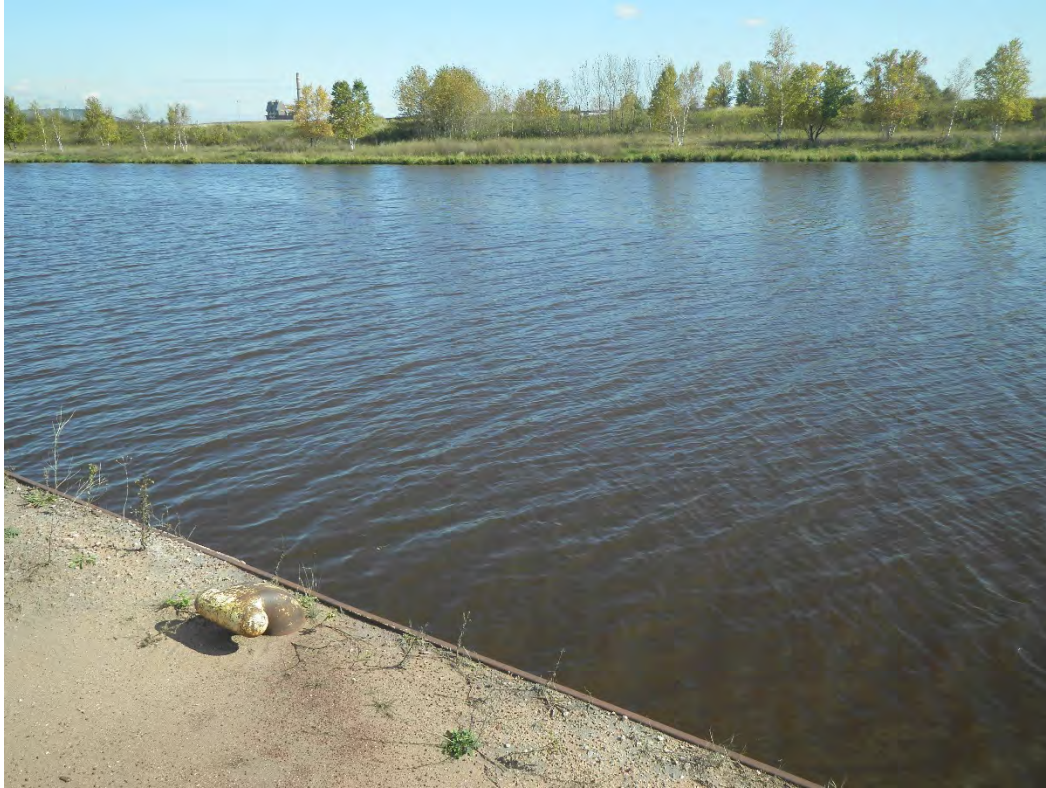
Location 8, Central dock wall along Slip 6/CAD, 50°
