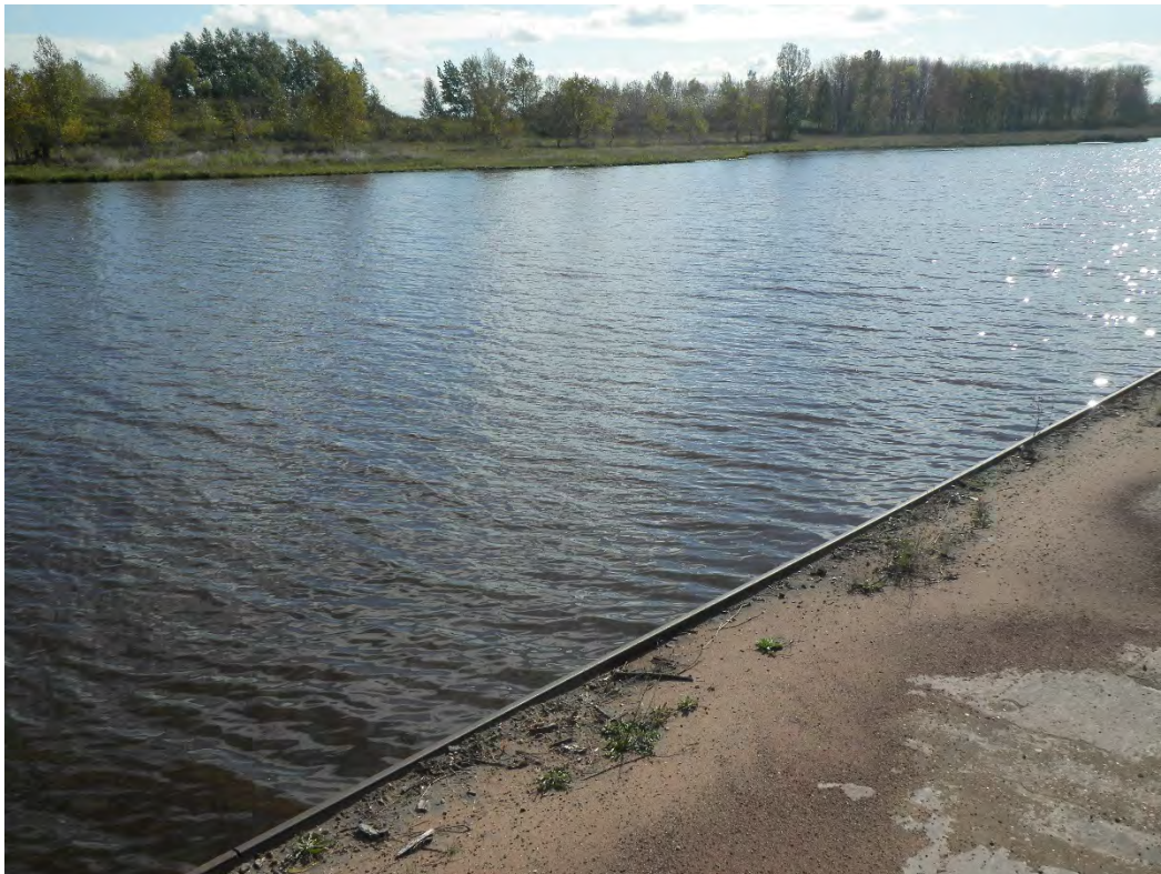
Location 8, Central dock wall along Slip 6/CAD, 130°
