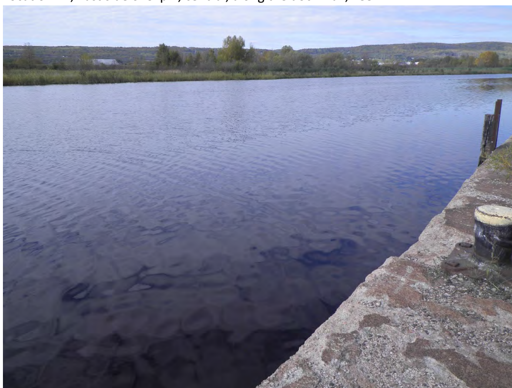
Location 24, East side of Slip 7, central, along the dock wall, 330 0
