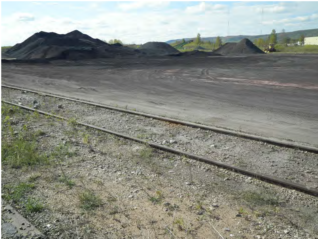
Location 9, Central dock wall along Slip 6/CAD, 215°
