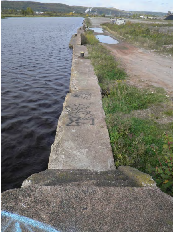
Slip 7 dock wall, view north from SW corner
