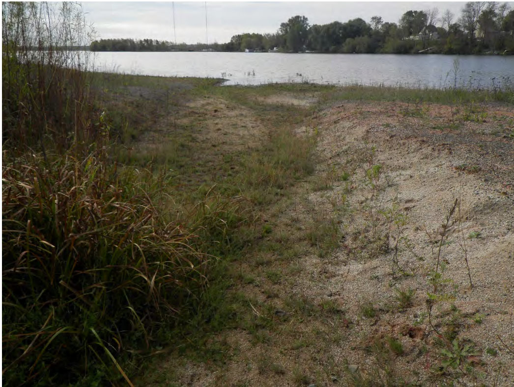
Stryker Bay, north end cap erosion
