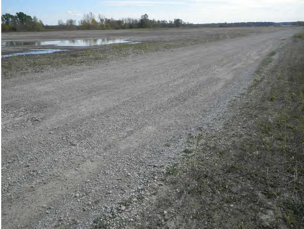
Location 23, East side of Slip 7, central, along the dock wall, 145 0
