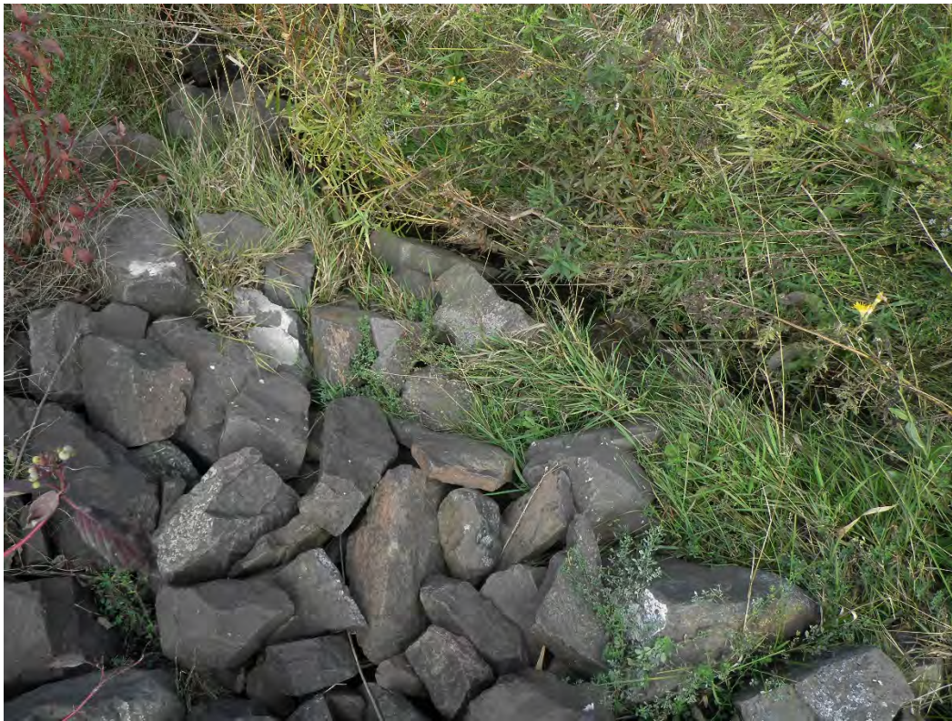
Stryker Bay, north end, French drain with channel outside
