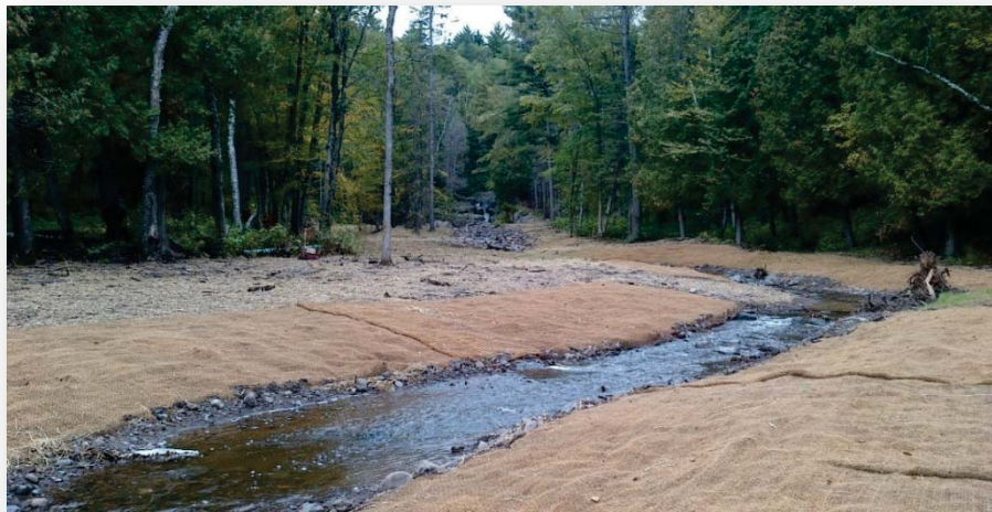
Restoration at Knowlton Creek. Photo credit: MNDNR.
