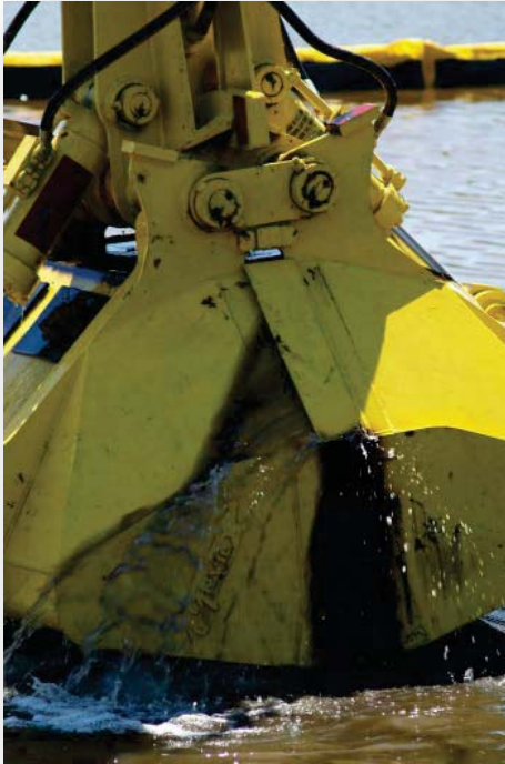
Dredging at Stryker Bay. Photo credit: MNDNR.
