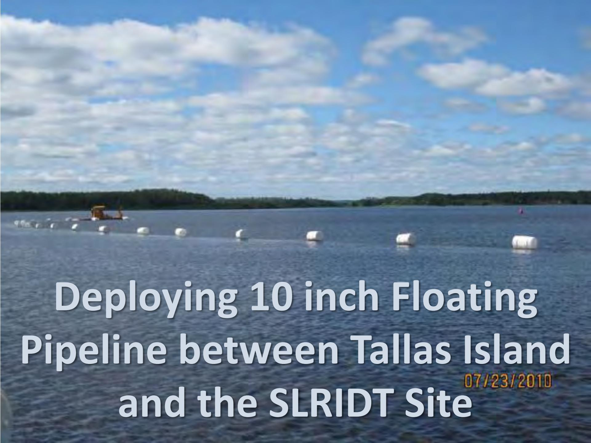
A photograph of a lake under a blue sky with scattered white clouds. In the foreground, a boat with a yellow canopy is positioned on the left, connected to a long, floating pipeline system. The pipeline consists of a series of white, cylindrical buoys connected by a dark line, stretching across the middle of the frame. The water is a deep blue. In the background, a dense forest line is visible across the lake, and the horizon is flat.
