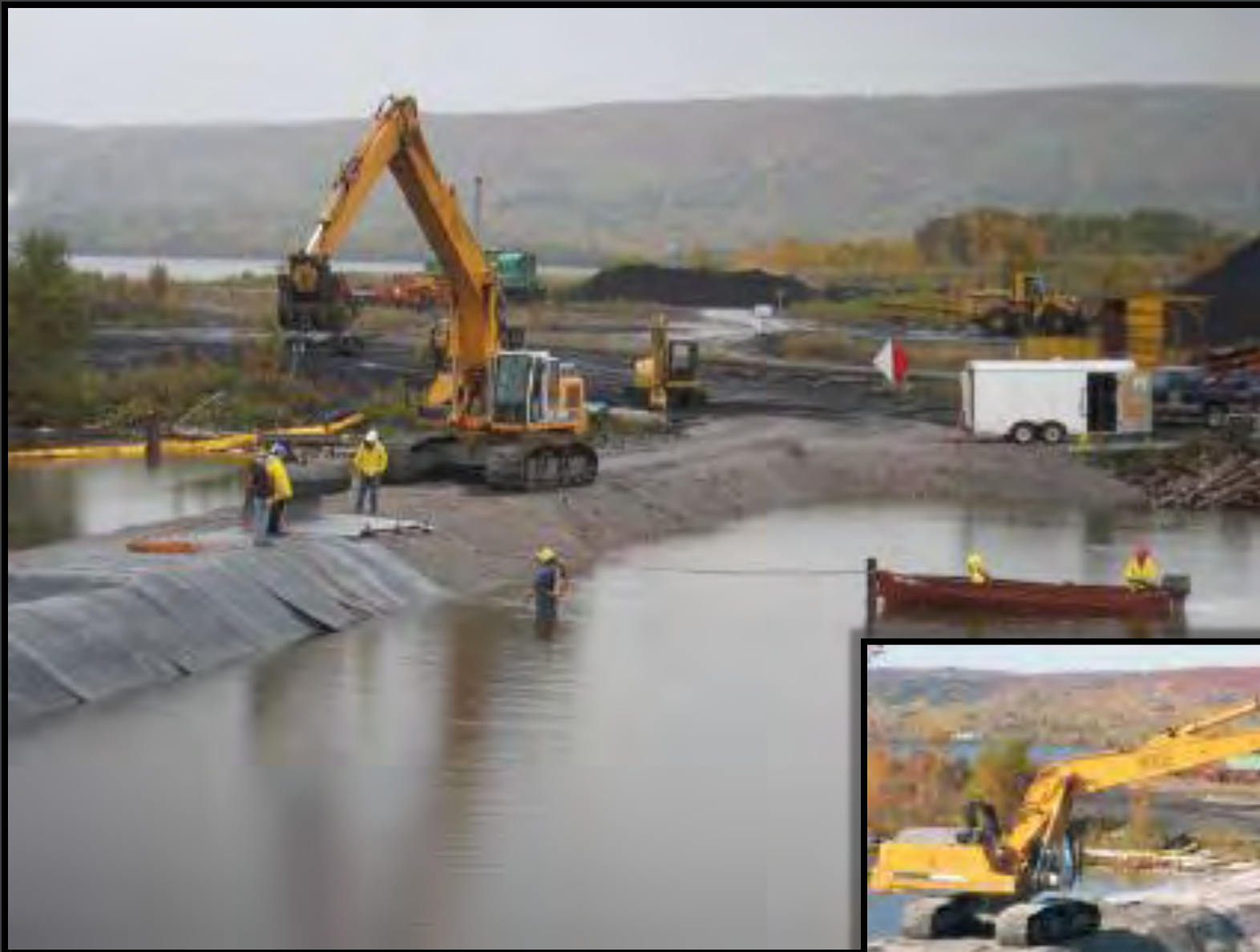
Clay Mat & Ballast Installation
