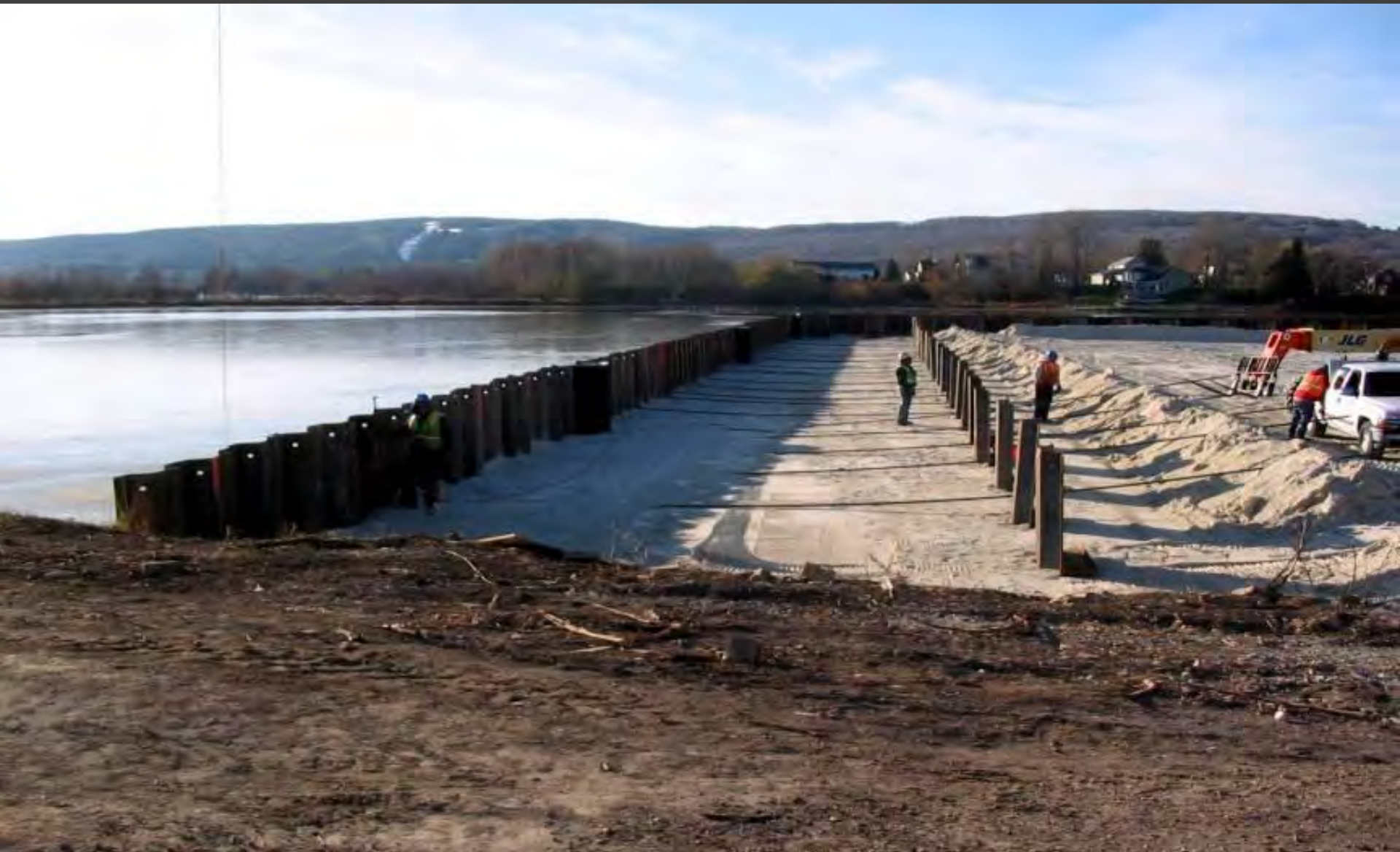
Installing Sheet Pile Wall Tie-backs
