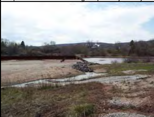
18: Area A. French Drain and outfall and/or spring flowing into surcharge cap and Stryker Bay
