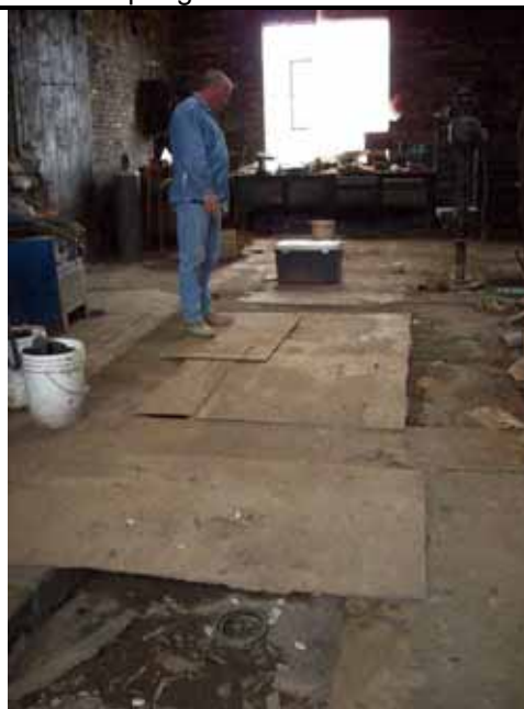
10: May 9, 2008. Area E, southern building on EBI property. Wood covering pit filled with approximately 1 foot of water over tarry material.
