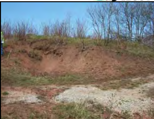
16: Area A. City storm sewer outfall from Fremont Avenue and resulting erosion. November 2006 – French drain installed to correct erosion problems in the surcharge cap in Stryker Bay.
