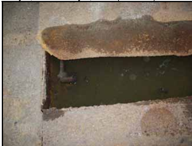
11: May 9, 2008. Area E, southern building on EBI property. Approximately 1 foot of water over tarry material in pit.
