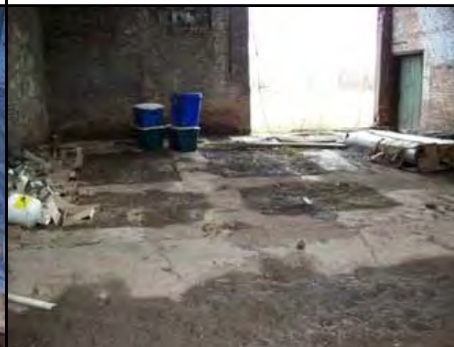
14: May 9, 2008. Area E, south-eastern building on EBI property. Openings in concrete floor filled in with soil.
