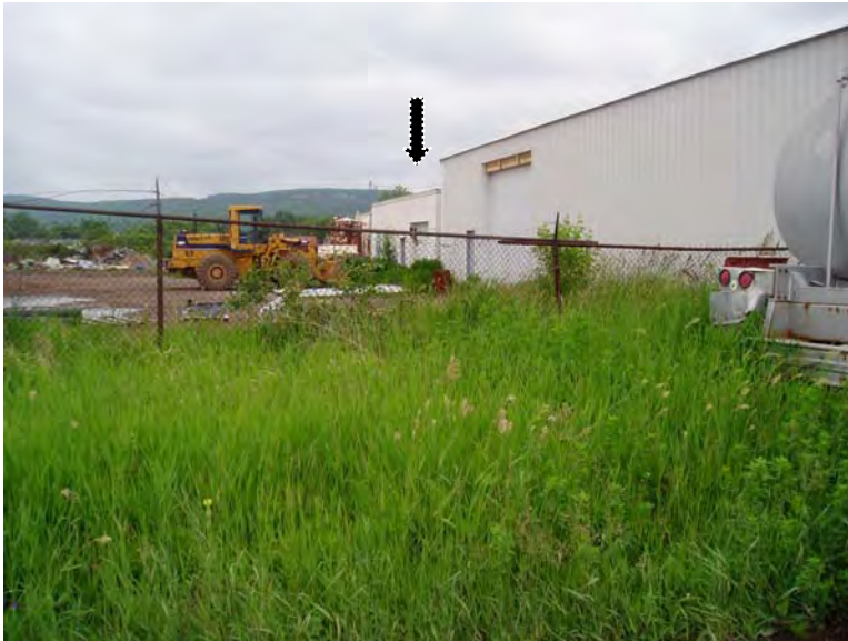
Represented by the arrow is the south side of former Duluth Auto Wrecking Inc. where residual contamination remains.
