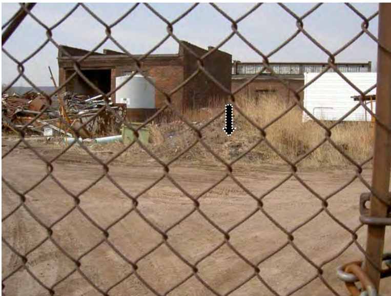
Looking west from the east side of Area E, this pile, excavated during gas line installation, reportedly contains coal tar.
