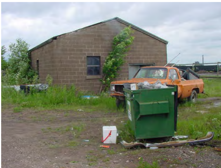
Residual Contamination is present under this pump house in Area D.
