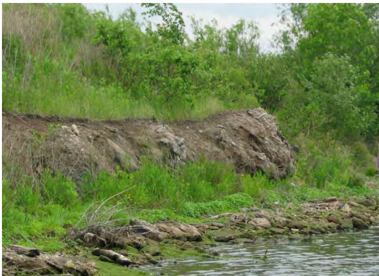
Erosion was observed along the west shore of the 59 th Avenue peninsula. The location was marked using GPS and is shown as Area F 1 on Figure 7
