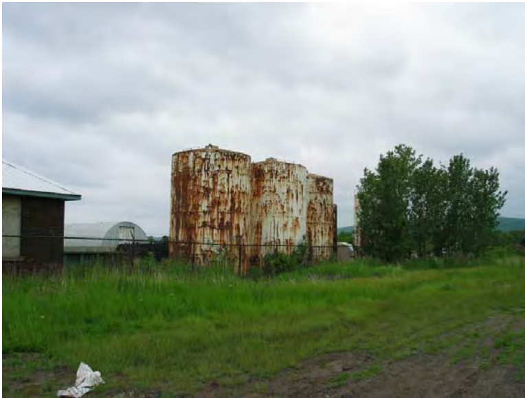
Shown to the left is the north side of Area E looking to the southwest.
