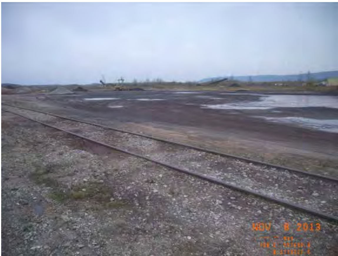
Location 9, Central dock wall along slip 6/CAD, 215°
