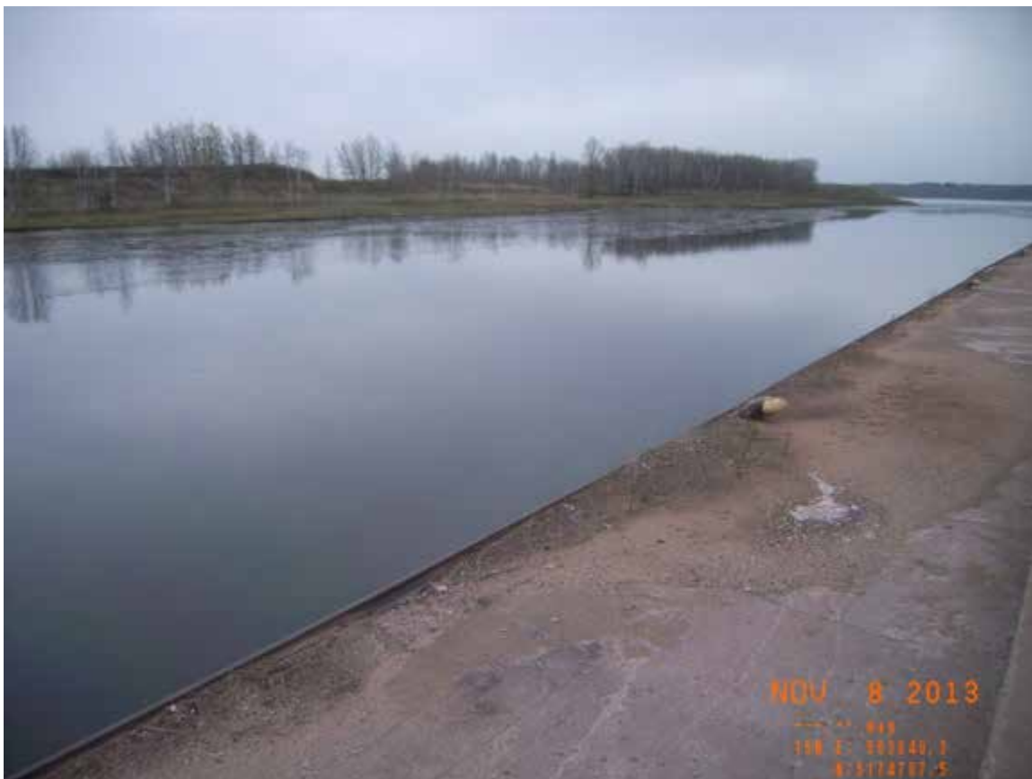
Location 8, Central dock wall along slip 6/CAD, 130 0
