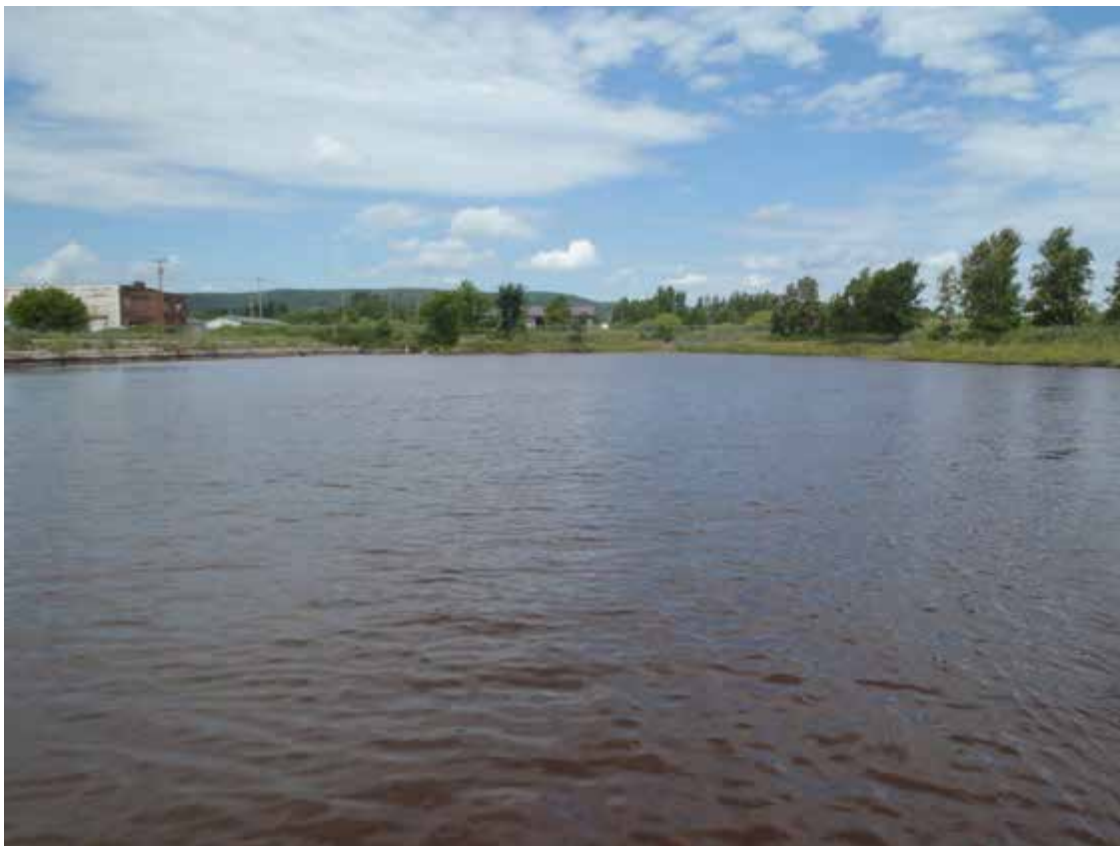
Photo 3 – Slip 6, north end, view north
