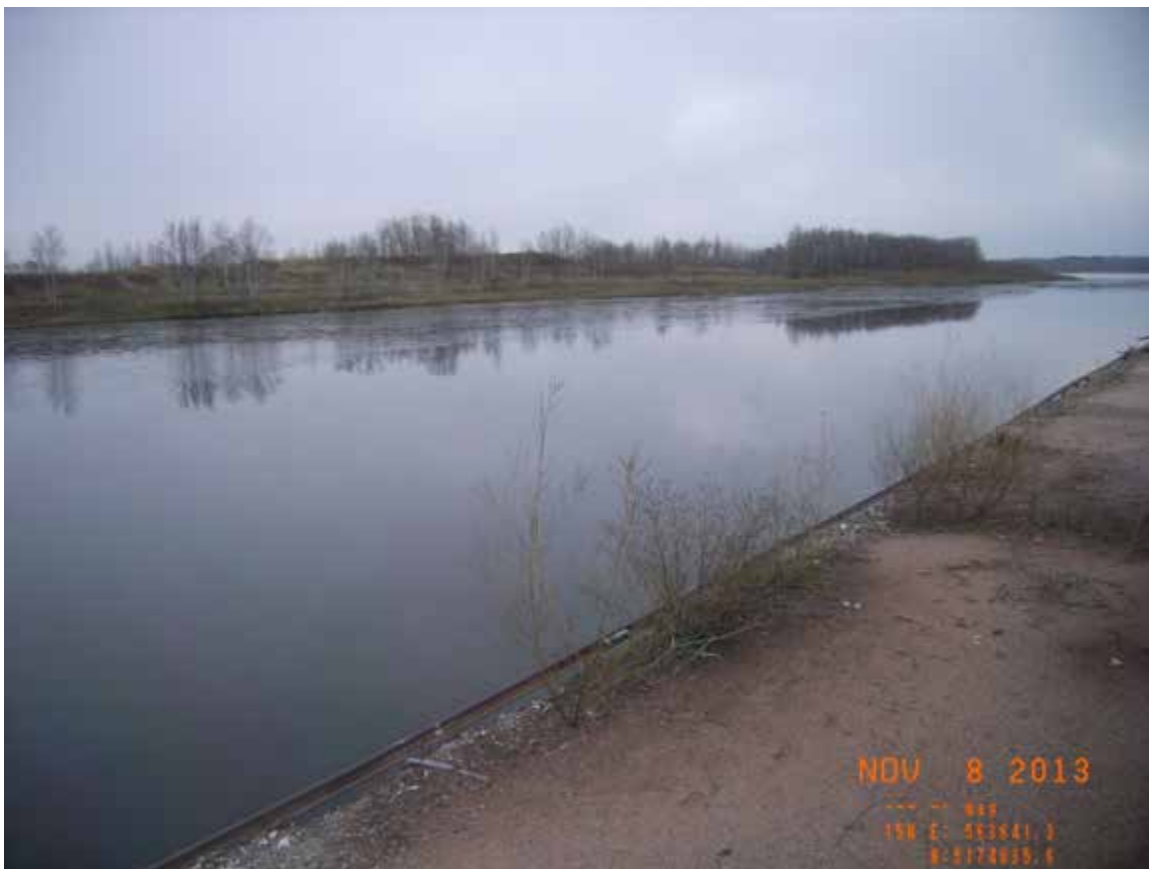
Location 9, Central dock wall along slip 6/CAD, 145°
