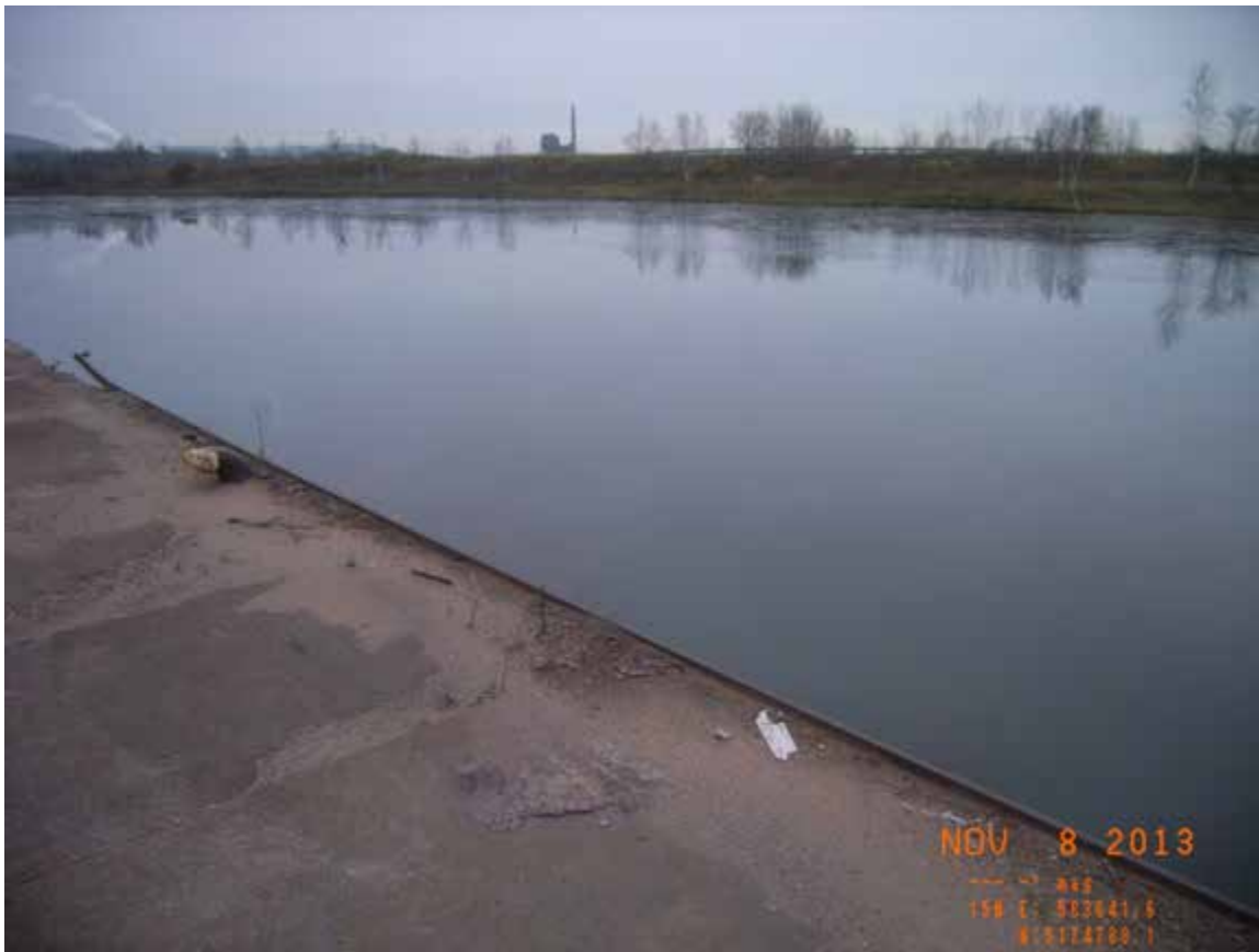
Location 8, Central dock wall along slip 6/CAD, 50 0
