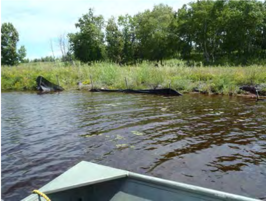
Photo 9 – Eastern shore of CAD, example of silt fence conditions
