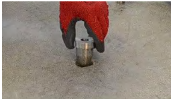
Figure 3. Installing the Drilling Guide.
