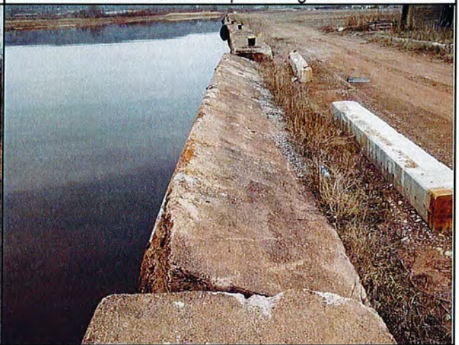
23: SedOU: Slumping of dock wall on slip 7.
