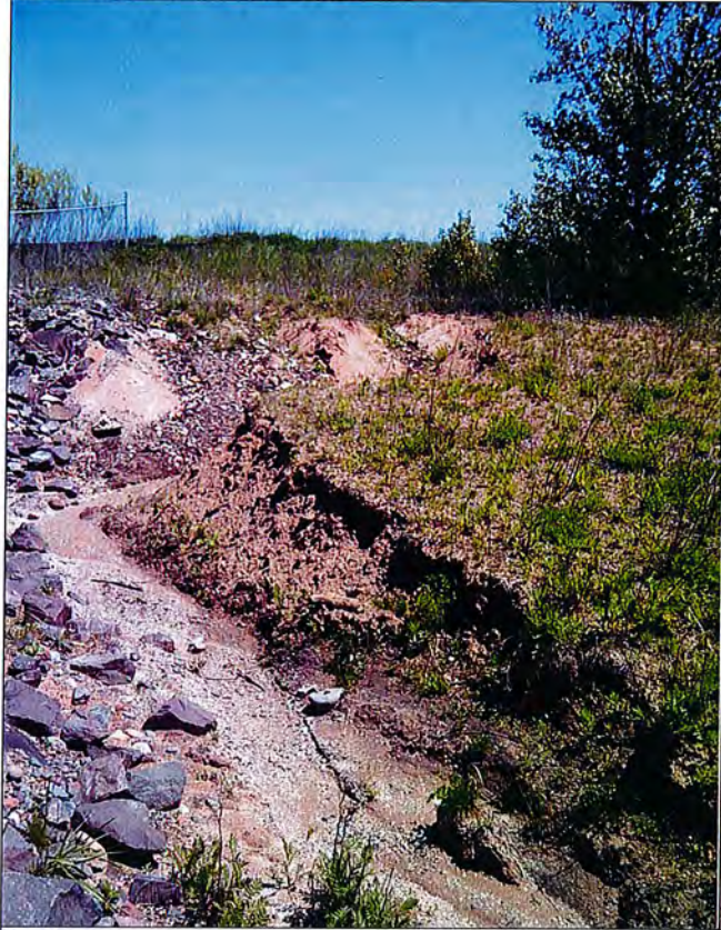
28: New erosion channel forming around repairs at NE corner of Slip 6.
