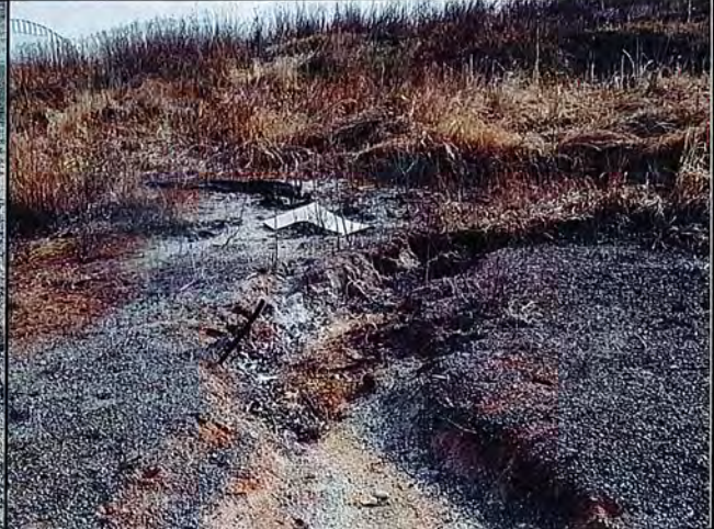
5: SedOU: Erosion of native material near Stryker Bay cap.
