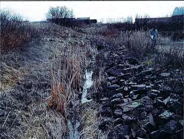
7: SedOU: City storm water diversion channel near NE corner of Stryker Bay cap, good condition.
