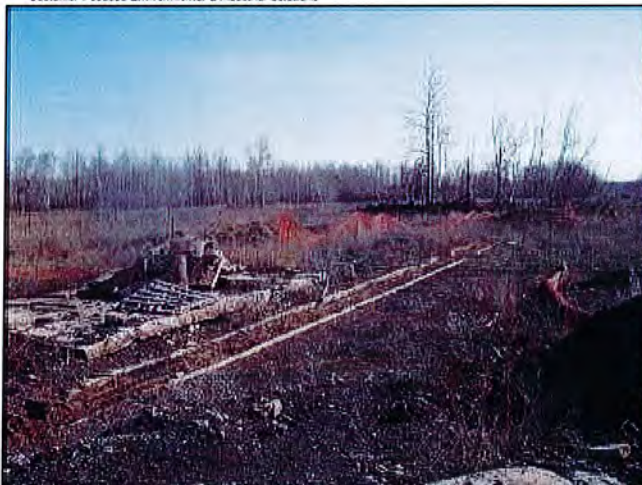
1a: OU-A: Tar soil removal from T-1 through T-4 area; clay applied to prevent erosion.
