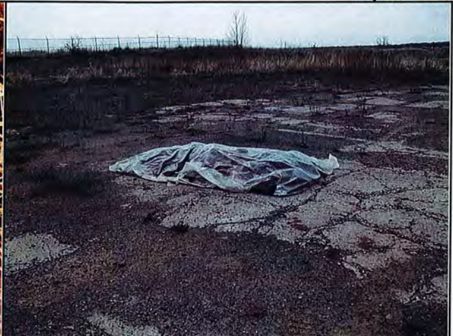
16: SOU Area A: Soil spoils pile, covered by plastic.
