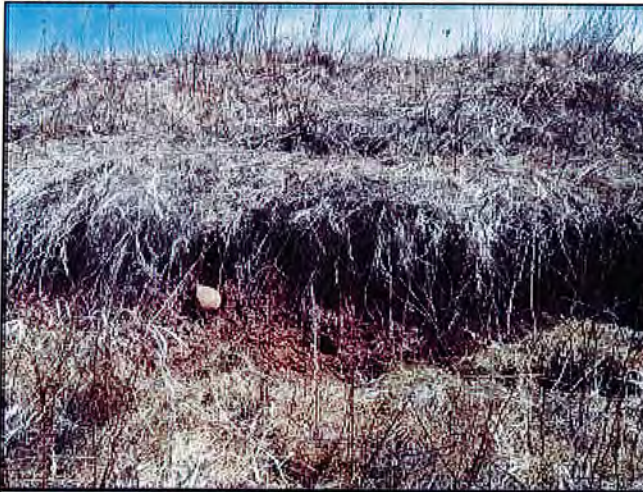
16: OU-J: Approximately 3' of slumping noted on cap/sidewall
