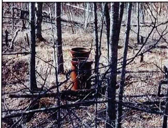
29b: Other AOC: Coke plant settling basin, sewer outfall history unknown, upright clay duct
