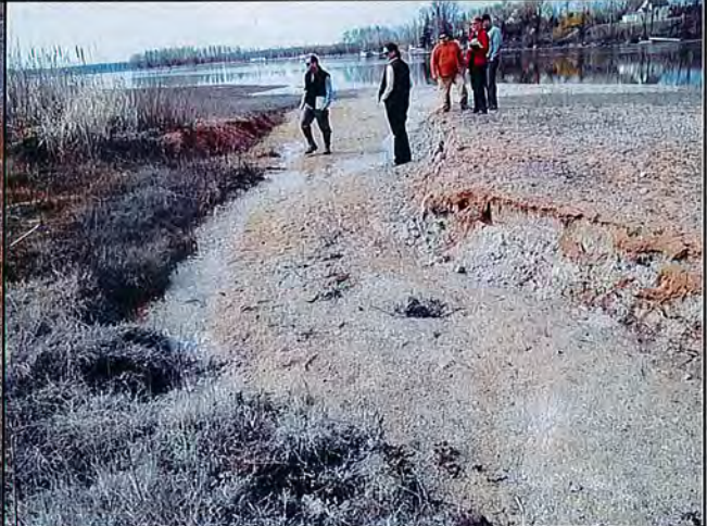
6b: SedOU: Erosion noted in water channel flowing onto Stryker Bay cap - riprap needed.
