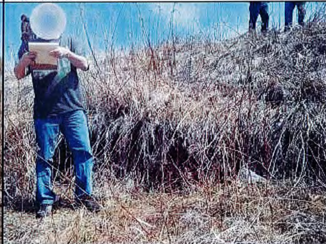
16: OU-J: Approximately 3' of slumping noted on cap/sidewall.
