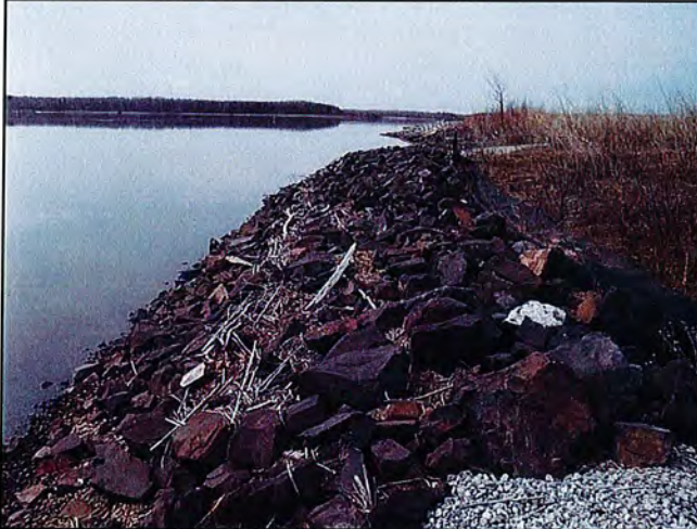
9b: SOU: Looking down slip 6, minor slumping
