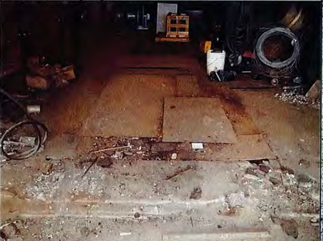
18: SOU Area E: Pit inside Terry Andersen building filled with up to 9' of tar.
