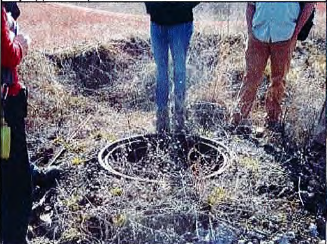
2b: OU-A: Manhole north of T-1 through T-4 area – no lid.
