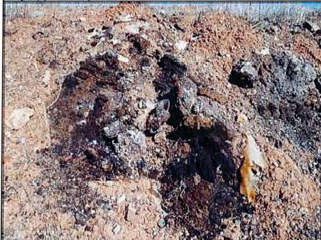
1c: OU-A: Tar soil removal from T-1 through T-4 area; clay applied to prevent erosion.
