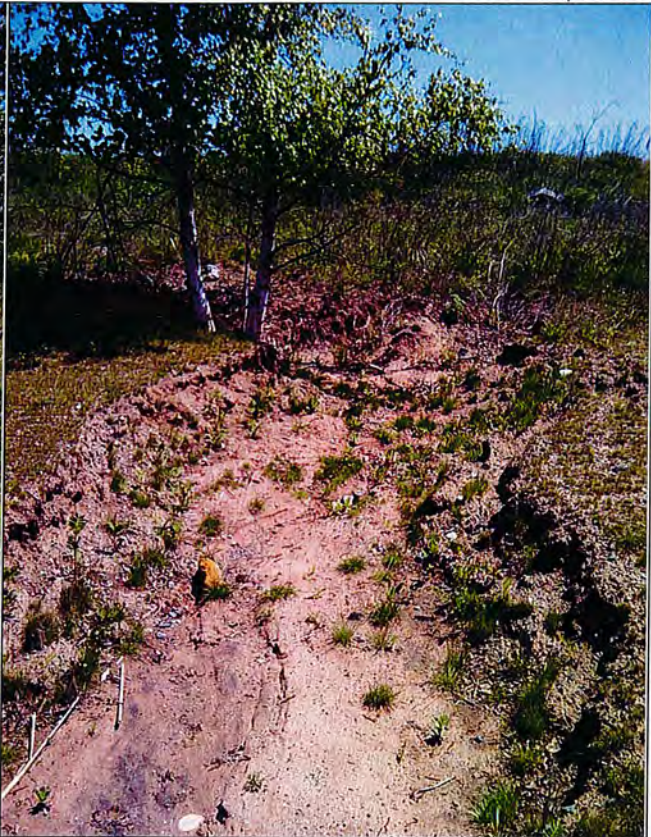
29: Erosion into cap along east side of Slip 6 (Area C).
