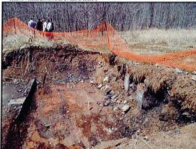
14a: Excavation of soils, fences down near Coke Oven Battery Foundation.
