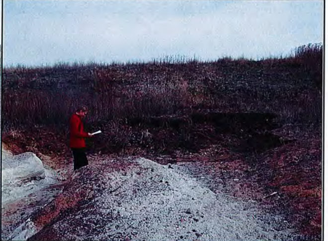
3b: SedOU: Significant erosion noted in native material near cap
