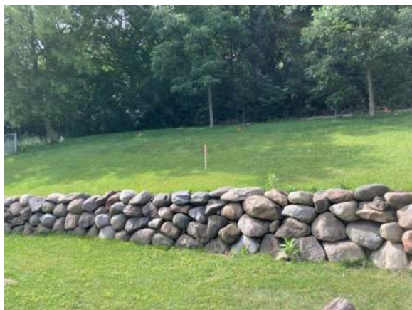
Rock retaining wall at 642
