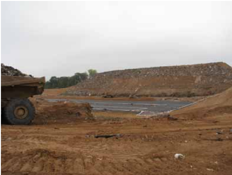
Contractor moving waste (~10/5/09)
