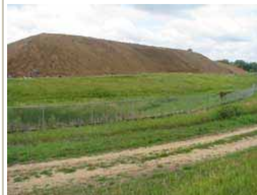
Waste stockpile is covered with soil on the north side of site.
