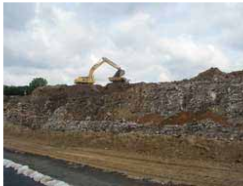
Contractor is completing waste move from first cell.
