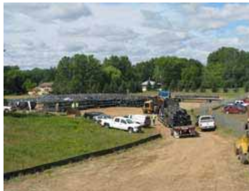
Liner rolls stockpiled on site.
