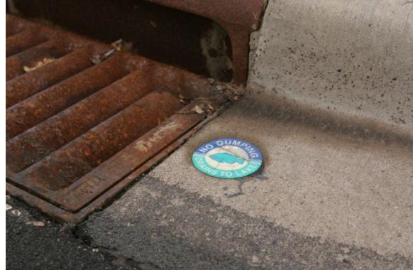
Storm sewer lines are usually constructed with "push-on" joints and are not normally watertight unless they are built in an area where the water table is high. This means that petroleum entering the sewer from the surface can seep out of the sewer line into the bedding material and surrounding soil. Conversely, petroleum from leaking underground storage tanks can percolate through the soil surrounding the sewer line and enter it through the joints or seams.
