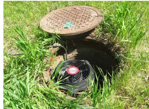
To power the fan, use an extension cord to a nearby outlet or generator. If possible, direct the exhaust away from passersby, buildings, and fresh-air intakes.
