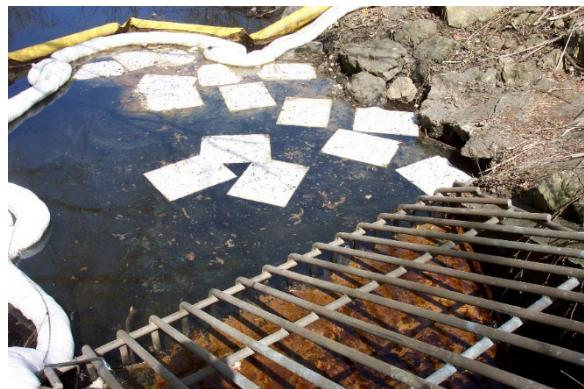
Once boom is in place, a controlled flush of the sewer can be done to collect the oil at the discharge point and further assess how much oil is present in the line. For a large volume of fuel in the sewer, it may be advisable to consider waiting to flush the line until a vacuum truck is on scene to recover the fuel.
