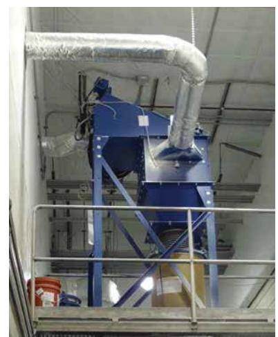
CPC-3 - Powdered milk dust in cheese factory 1,200 cfm (2,038 m³/h)
