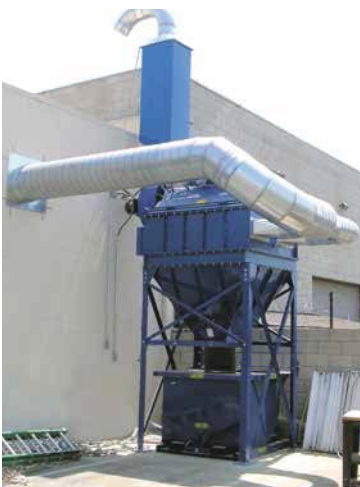
CPC-12 on Wood Dust at furniture manufacturer 7,000 cfm (11,891 m³/h)
