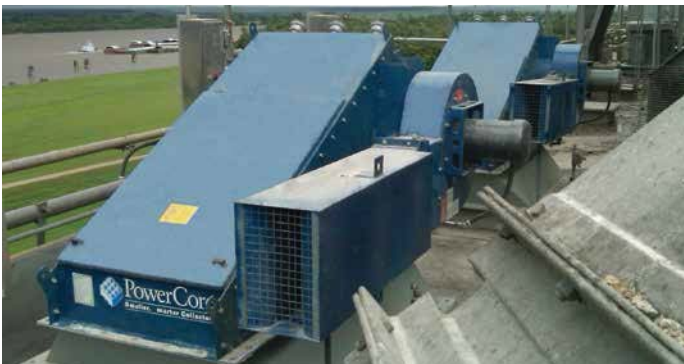
CPV-6 - Direct bin venting distributor head 2,400 cfm (4,077 m³/h)
