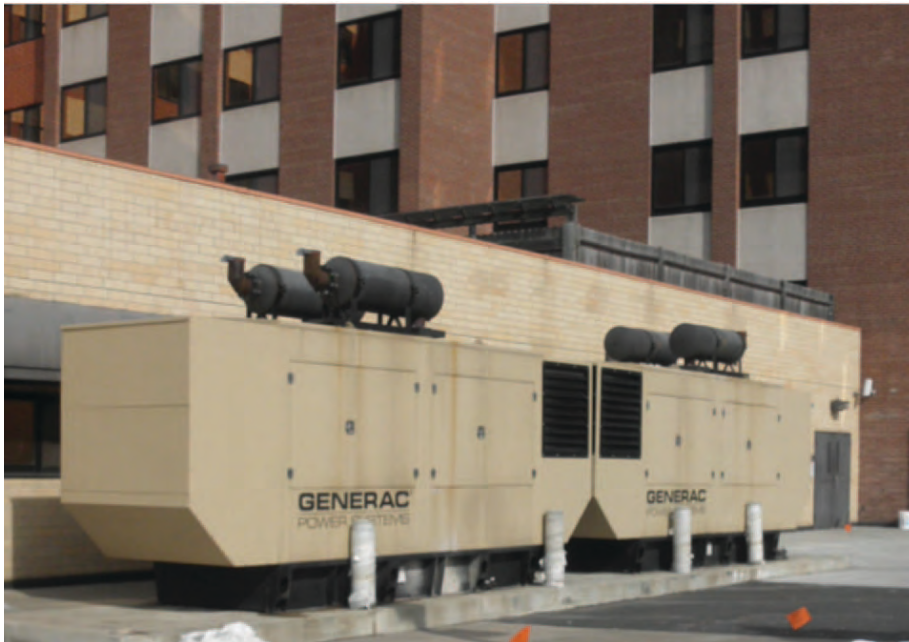
A typical diesel generator installation at a nursing home located near resident rooms. Low smokestacks result in poor air dispersion, and people can be exposed to exhaust through windows and building air intake vents.
