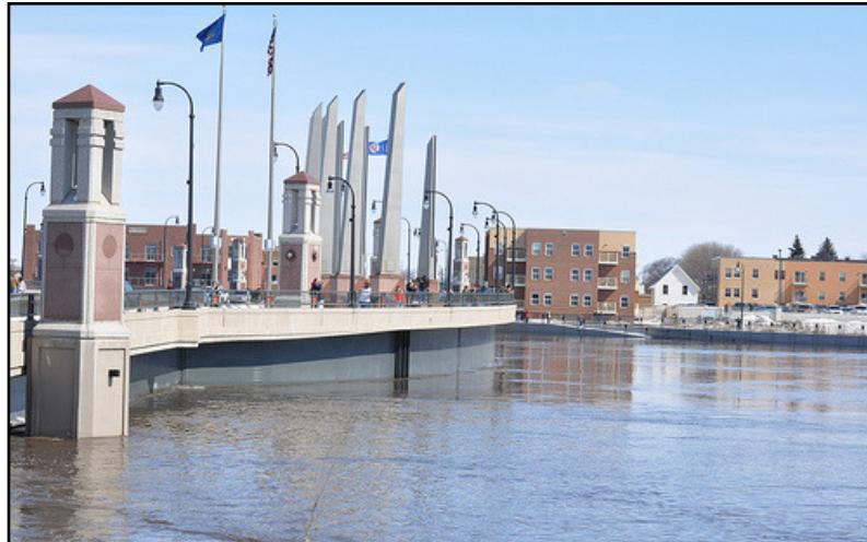
Main Avenue Bridge looking toward Moorhead from Fargo.
