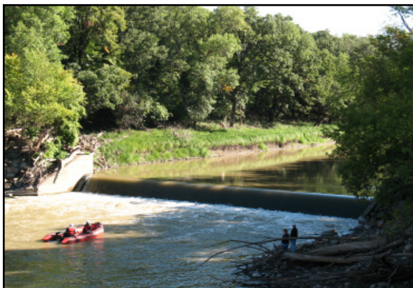
Hickson Dam before retrofit.
