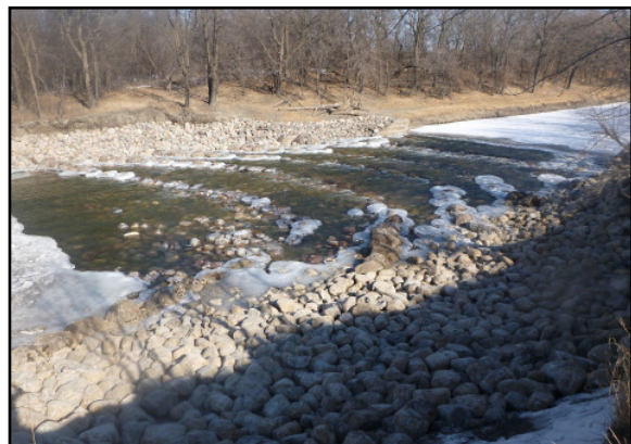
Hickson rapids, after dam retrofit.
