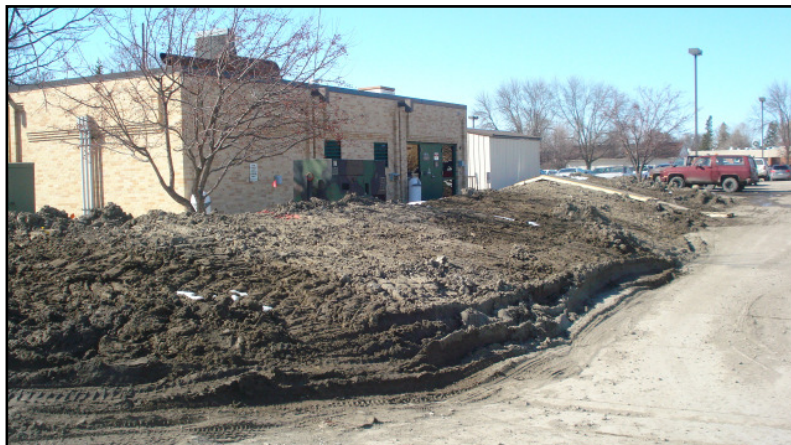
Dikes helped save many structures from incurring major flood damages.
