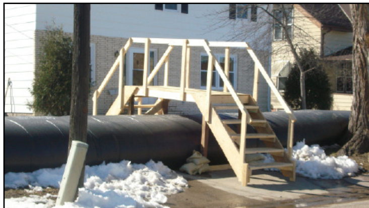
Allowing access to homes on the wrong side of a contingency dike involves building stairs over it. Moorhead, MN 2009.
