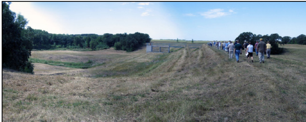
A dry dam, which only holds water during high-water periods.
