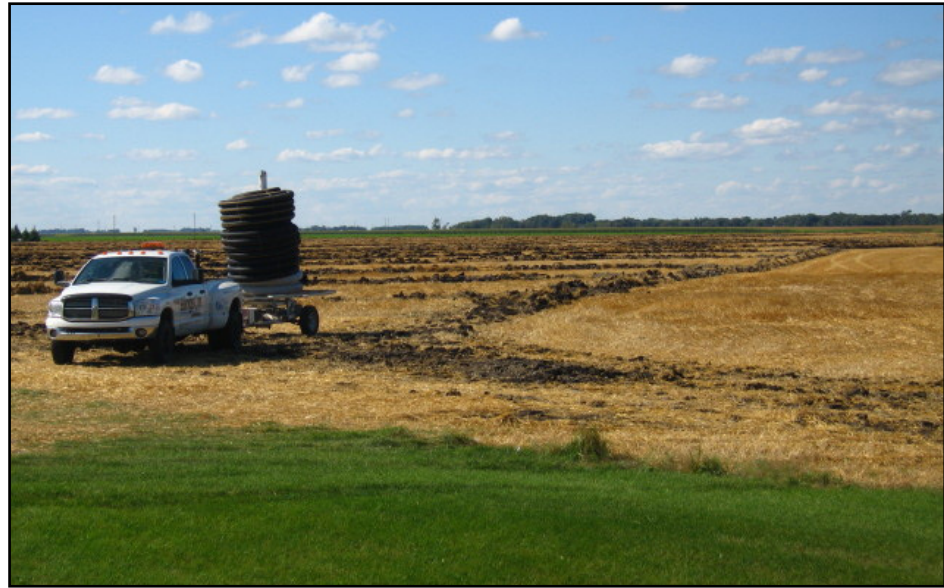
Installing plastic drain tile near Glyndon, MN.
