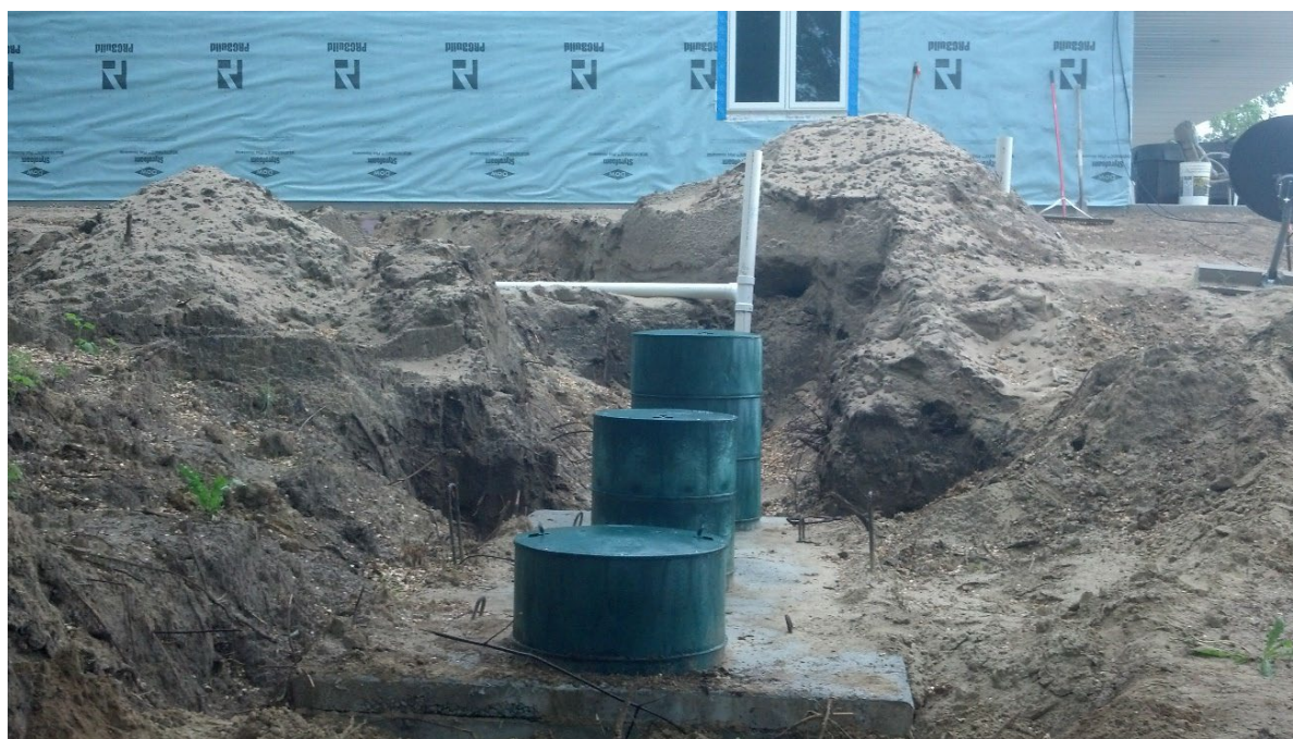
Figure 12. The installation of concrete sewage tank
