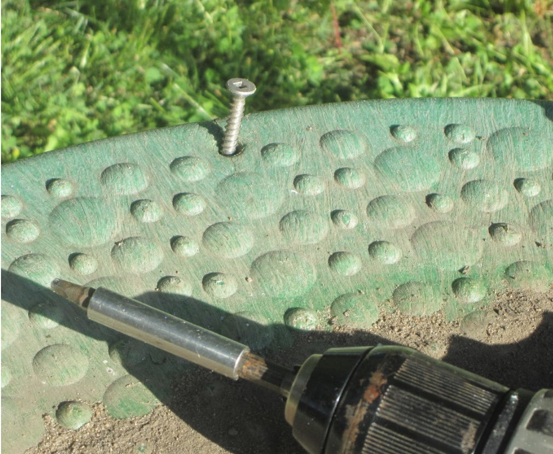
Figure 22. Maintenance hole covers identified as structurally unsound or unsecured are an ITPHS
