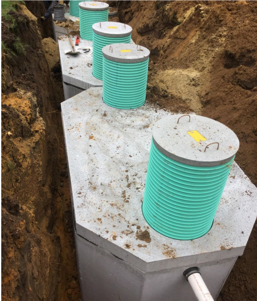
Figure 12. The installation of concrete sewage tanks
