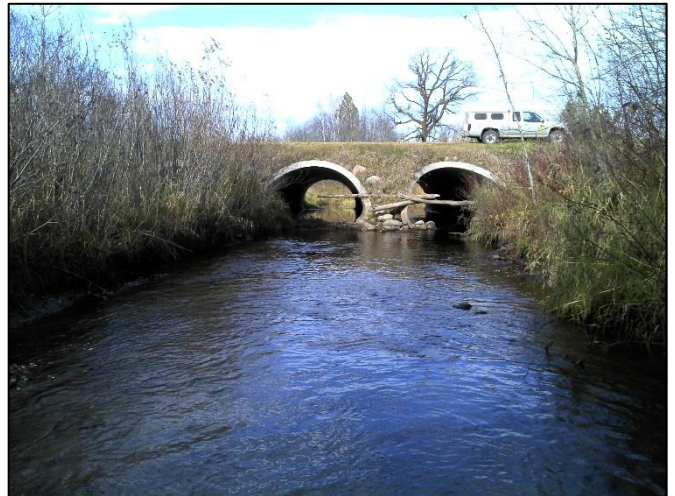
Figure 47. Site 12RN010 culverts (photo taken on 10/20/15).
