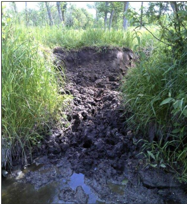
Photo 7. Close up of bank erosion on Darrigan’s Creek caused by cattle accessing the creek.
