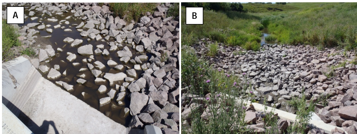
Photo 6. The channel a short distance below the biological site. A) On the upstream side of CR 33. There was only a minimal amount of standing water in the channel. B) On the downstream side, there is high gradient within the new, rip-rapped stream bed.
