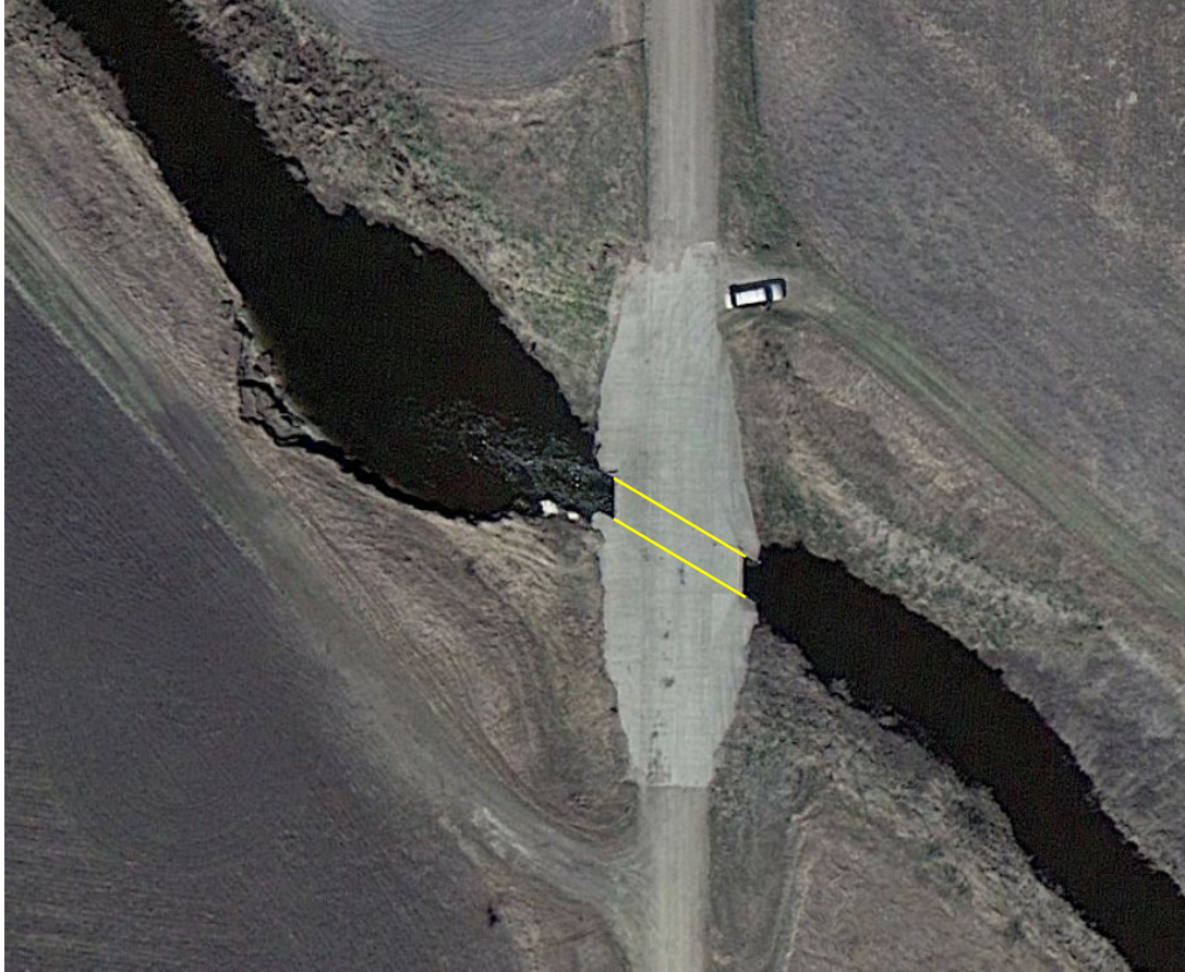
Figure 29. Culvert on Twp. Rd 105. The culvert is undersized, creating an increase in water velocity (note the water turbulence on the downstream (left) side of the culvert), and the associated eroding banks, especially the west bank. Note that the field access road will soon be impacted. The yellow lines show the culvert width, which is much narrower than the channel width.
