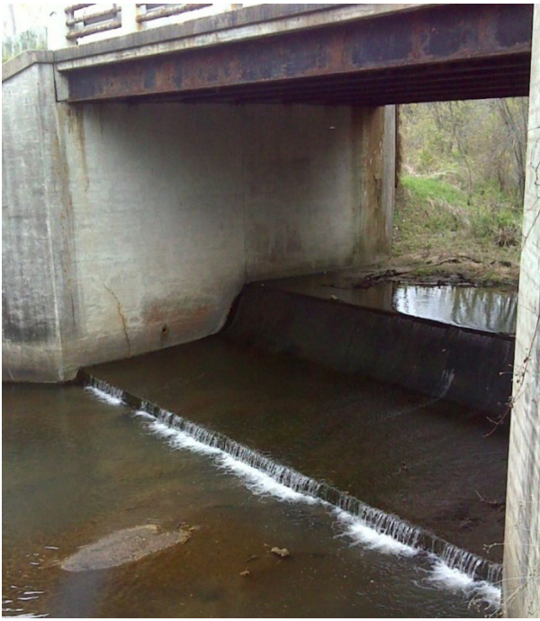
Figure 100. Dam under Highway 42 Bridge, downstream from 10LM030 (0.2 miles). Estimated 2 ft of vertical drop.
