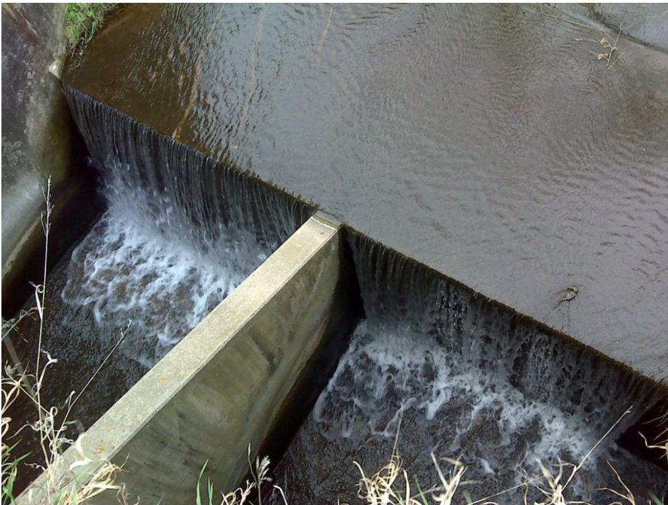
Figure 101. Dam by culvert under Highway 61 Bridge, downstream of 10LM030 (~1 mile). Estimated 6 feet of vertical drop.
