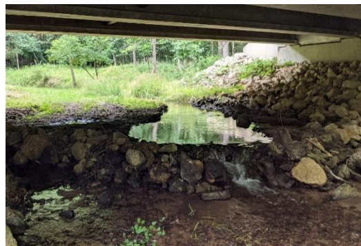
Figure 12: Rock dam below CSAH 21 in Trout Brook.
