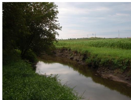
Figure 154. Bank erosion at site 14MN038 (September 3, 2014)
