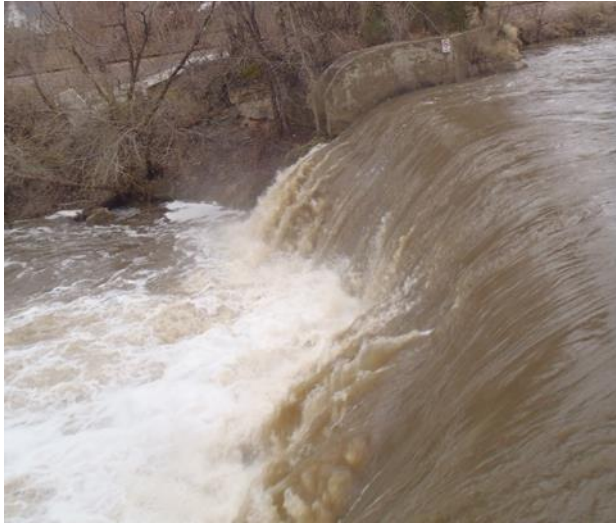
Figure 201. Sand Creek dam
