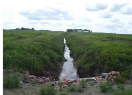
Figure 37. Site 14MN068 (July 16, 2014)
