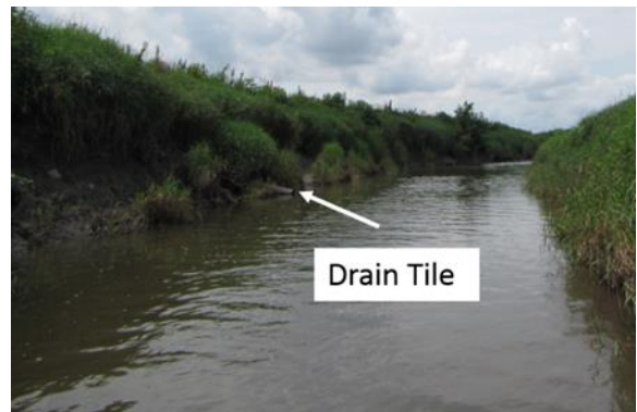
Figure 8. Drain tile at site 14MN067 (August 3, 2016)
