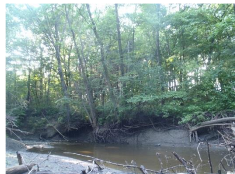
Figure 208. Bank erosion at site 14MN129 (July 28, 2014)
