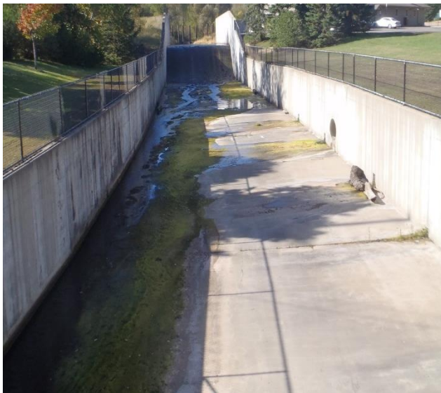
Figure 305. Artificial channel constructed on Chaska Creek downstream of site 00MN010 (September 30, 2013)
