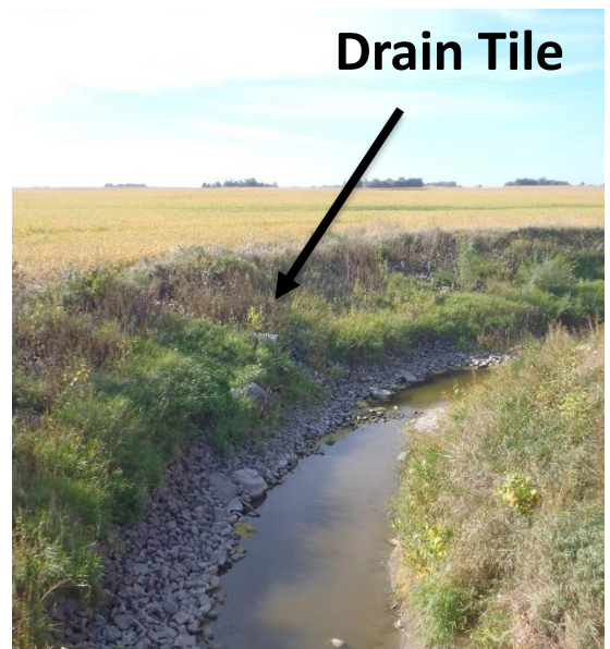
Figure 58. Drain tile at site 14MN052 (September 30, 2013)
