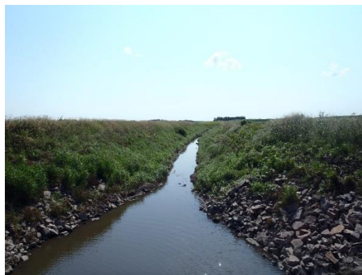
Figure 133. Lack of sinuosity at site 14MN089 (July 29, 20914)
