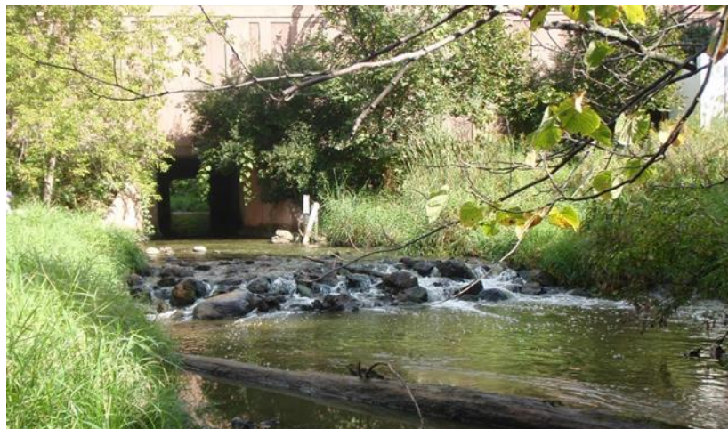
Figure 320. Rock dam downstream of dam
