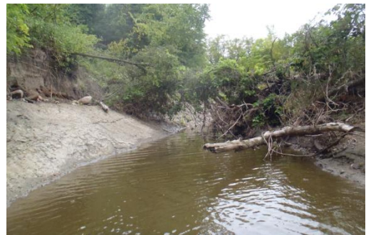
Figure 258. Bank erosion at site 14MN120 (August 28, 2014)
