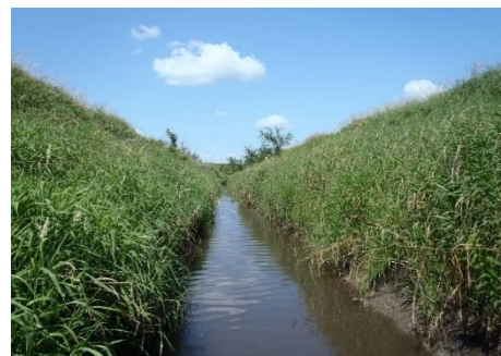
Figure 121. Lack of sinuosity at site 14MN088
