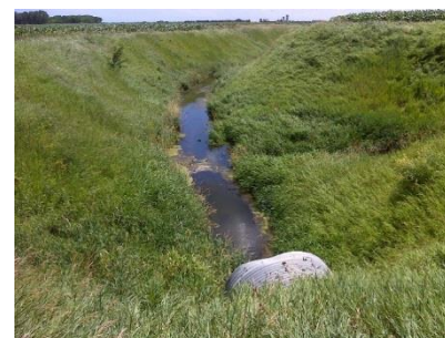
Figure 176. Site 14MN080 (July 5, 2016)
