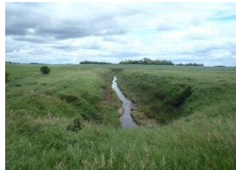
Figure 130. Poor sinuosity at site 14MN058.
