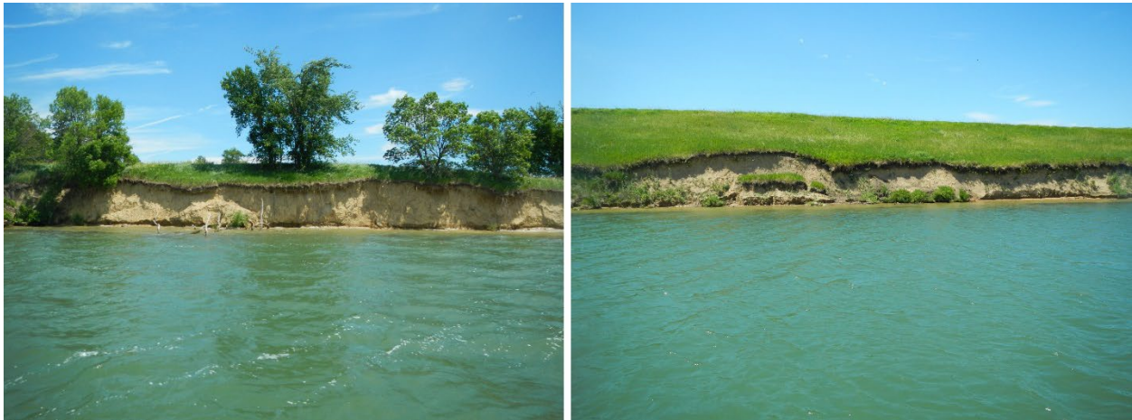
Figure 8. Examples of bank erosion present around East Twin Lake.
