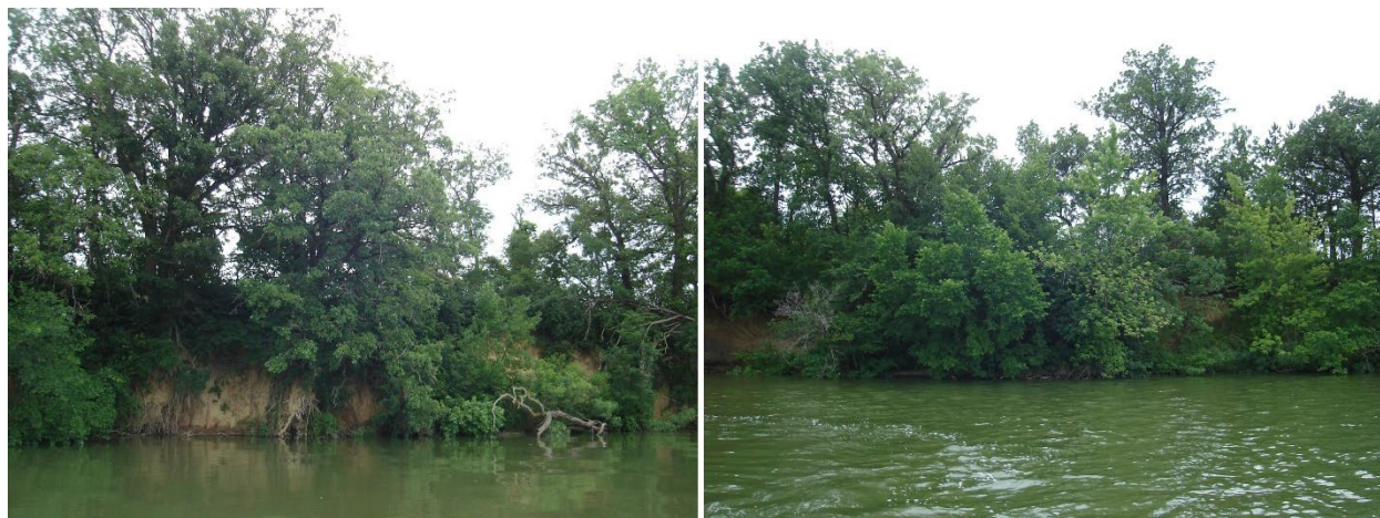
Figure 3. Examples of bank erosion present around Double Lake.
