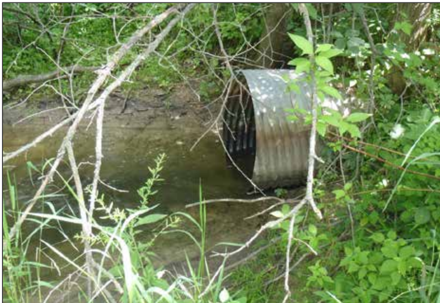
Photo 18. Downstream end of the culvert at Peloquin Avenue NW.
