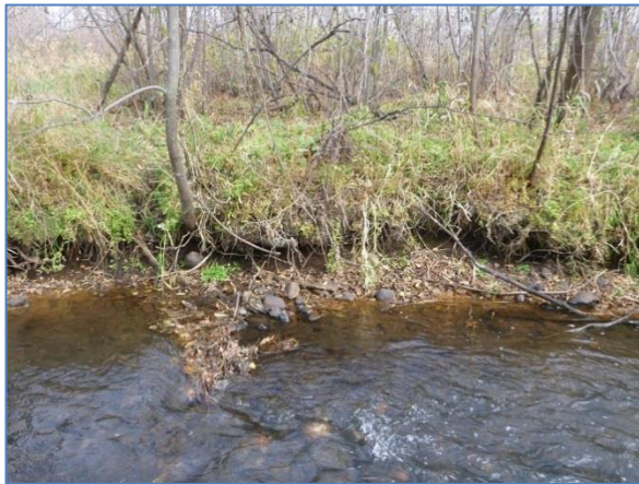
Figure 85. Bank erosion observed during geomorphic survey upstream of Nature Rd. on 10/21/2015.
