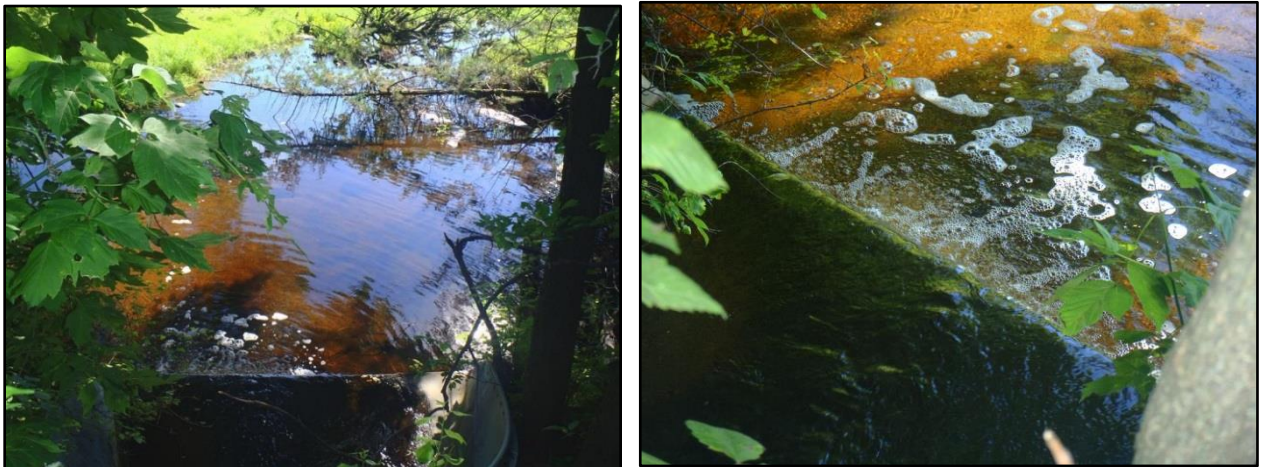
Figure 40. Outfall of Great River Rd. culvert. Photo taken 7/13/2018.
