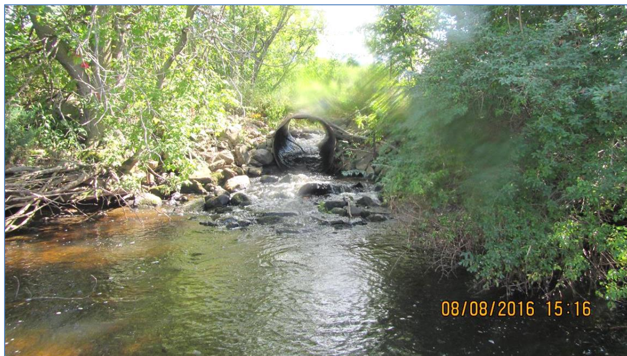
Figure 59. Private culvert on upstream end of 07UM101.
