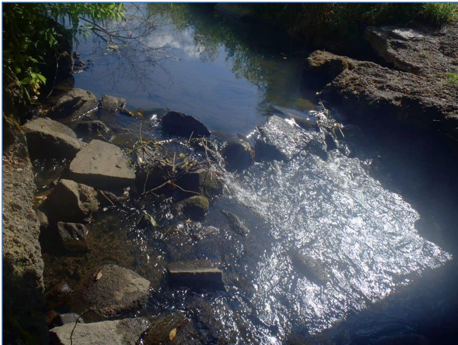
Figure 56. Artificial rock feature upstream of Stearns County CSAH75 crossing. Possibly for grade control.
