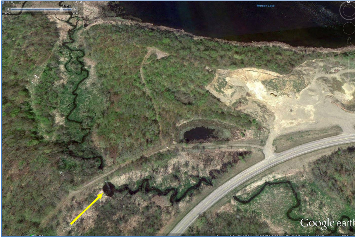
Figure 62. Private stream-road crossing, upstream of CR160 towards Merden Lake. Arrow points to evidence that the culvert is causing geomorphic instability. It is too small and causing a “fire hose” effect on the downstream side. Observed using Google Earth aerial imagery.
