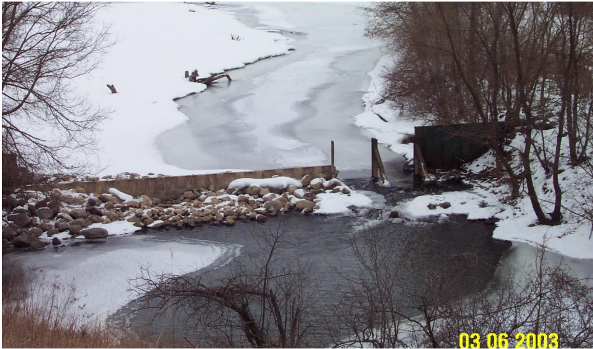
Figure 82. Pictures of the Sartell State Wildlife Management Area (WMA) dam on Little Rock Creek, showing the varying degree to which this structure is a barrier to fish passage depending on dam height, water level, and other factors. Photos courtesy of MN DNR.
