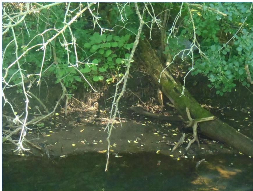
Figure 58. Bank erosion at downstream scour pool at outlet of Stearns County CSAH75 road crossing.
