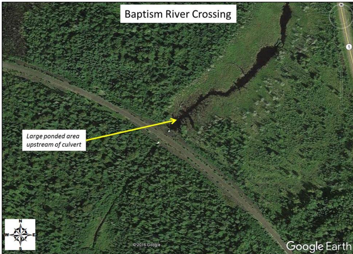
Figure 100. Aerial photo of the Baptism River RR crossing, showing large ponded area upstream of culvert.
