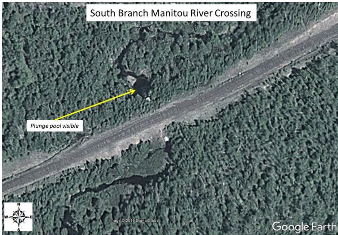
Figure 96. Aerial photo of the South Branch Manitou River RR lower crossing, showing plunge pool downstream of culvert.
