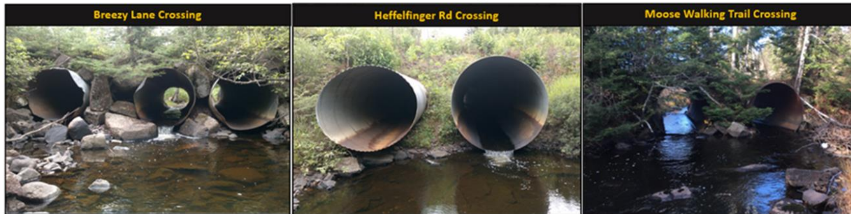
Figure 71. Profile of Hockain Creek generated with 1-m LIDAR elevation and watercourse data (top). Crossings of Hockamin Creek at three locations; Breezy Lane, Heffelfinger Rd, and Moose Walk Trail. The crossings at Breezy Lane and Heffelfinger Rd are barriers to aquatic organism passage and should be replaced.
