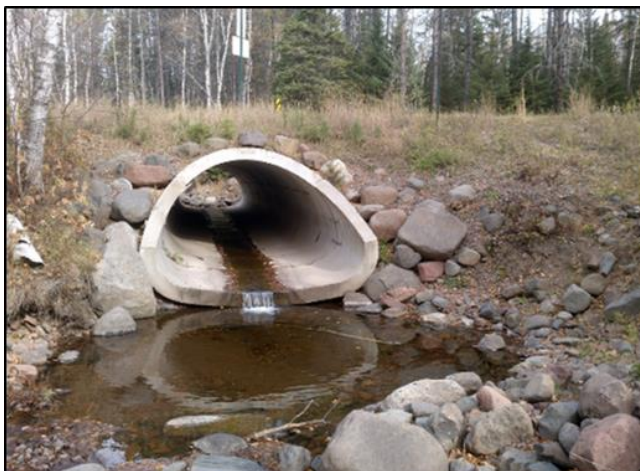
Figure 58. Woods Creek crossing under CR 58 crossing (left) and CR 60 (below). The CR 58 crossing is a barrier to fish migration and a priority for restoration.
