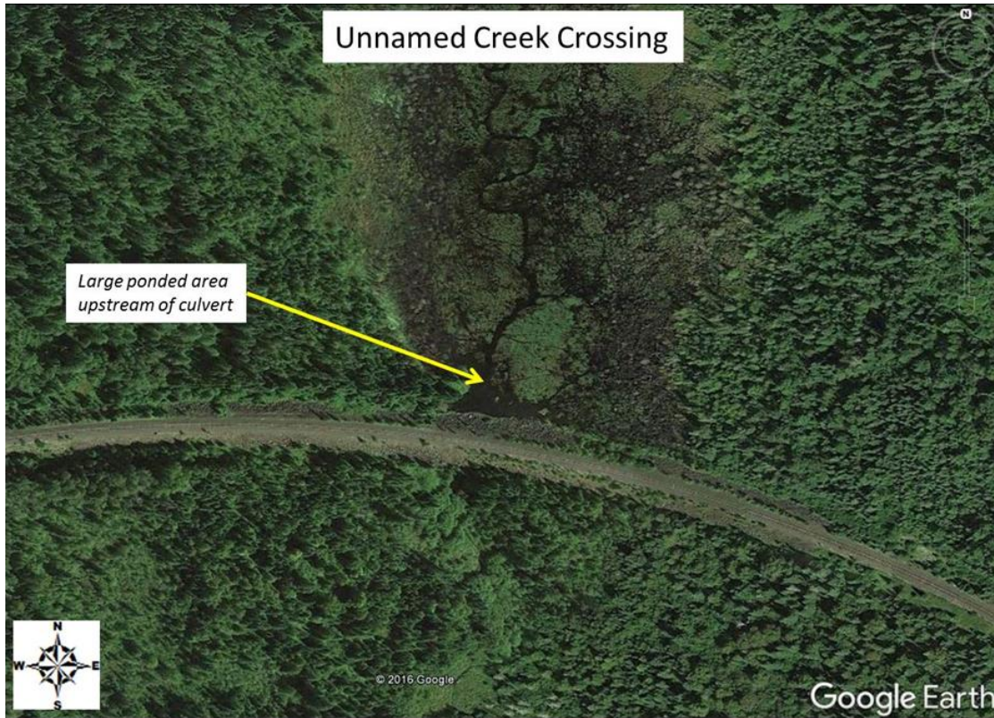
Figure 102. Aerial photo of the Unnamed Creek RR crossing, showing large ponded area upstream of culvert.
