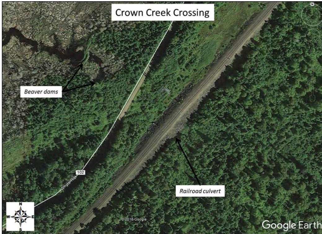
Figure 104. Aerial photo of the Crown Creek RR crossing. Crown Creek is difficult to see near the crossing.
