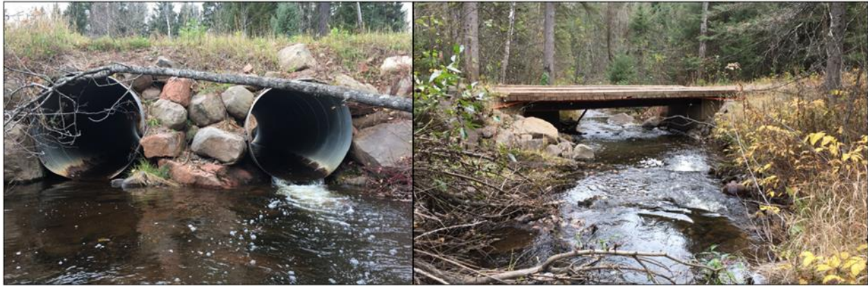
Figure 75. Perched and improperly set culverts at the Cooper Rd crossing create a partial barrier to fish passage (left), while a span bridge located just downstream allows full fish passage and helps maintain channel stability.
