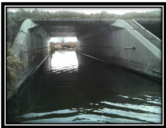
Figure 1 - Culvert on the Upper Iowa River
