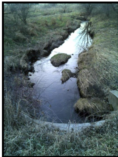
Figure 6 – Concrete arch culvert on 111 th avenue, Fillmore County
