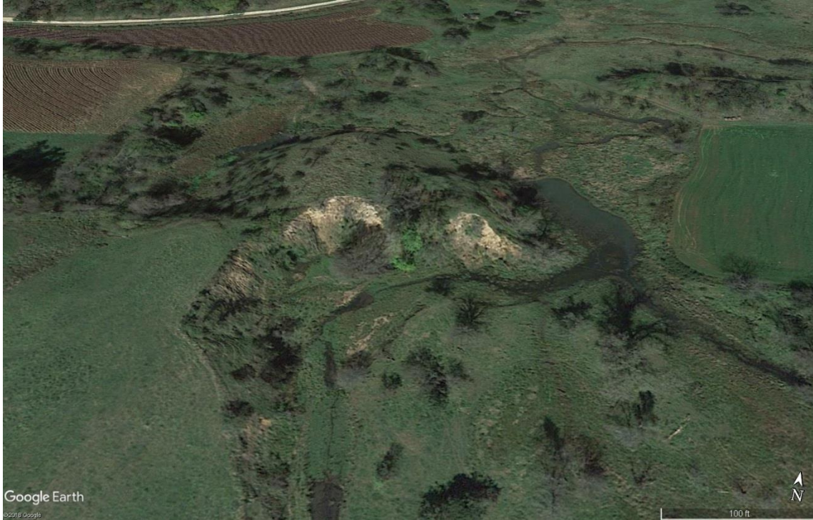
Figure 67. Eroding bank in catchment 18, looking downstream.
