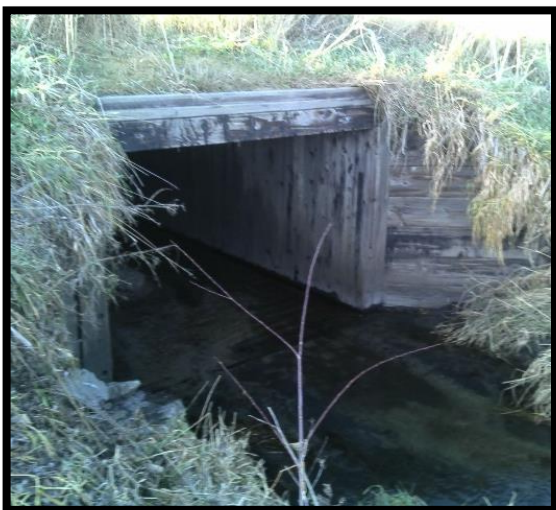
Figure5 – Wooden culvert on Fillmore County Highway 1
