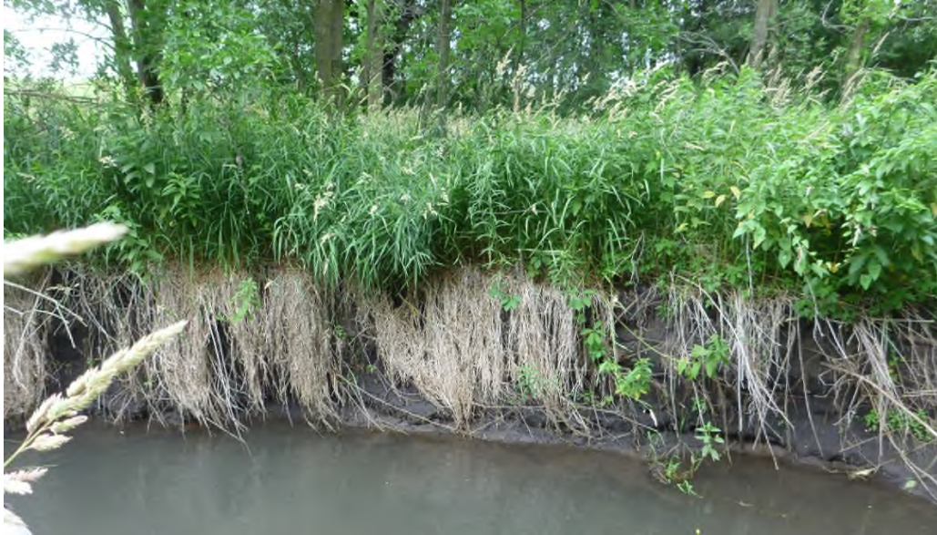
Figure 4. Eroding bank within the surveyed reach
