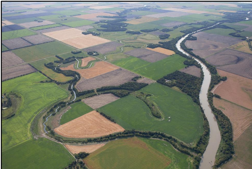
Figure 1-3. Aerial view of the completed Grand Marais Creek Outlet Restoration Project
