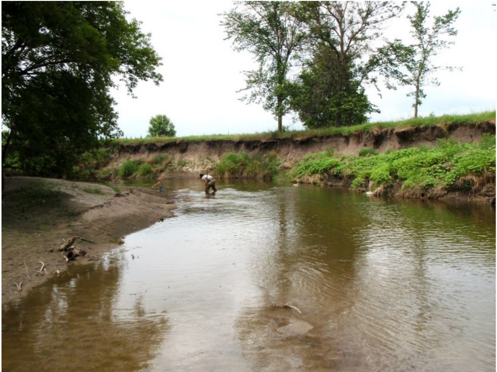
Figure 19. Severe bank erosion and excess sedimentation at Beaver Creek station 14DM014.
