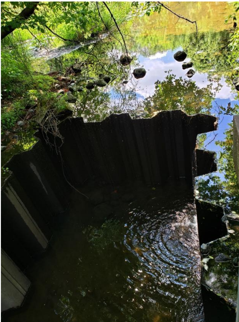
Figure 88. Dam structure downstream of Curtis Ave on Silver Creek.
