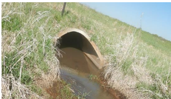
Figure 61. Culvert crossing off CR 11 in 2021.
