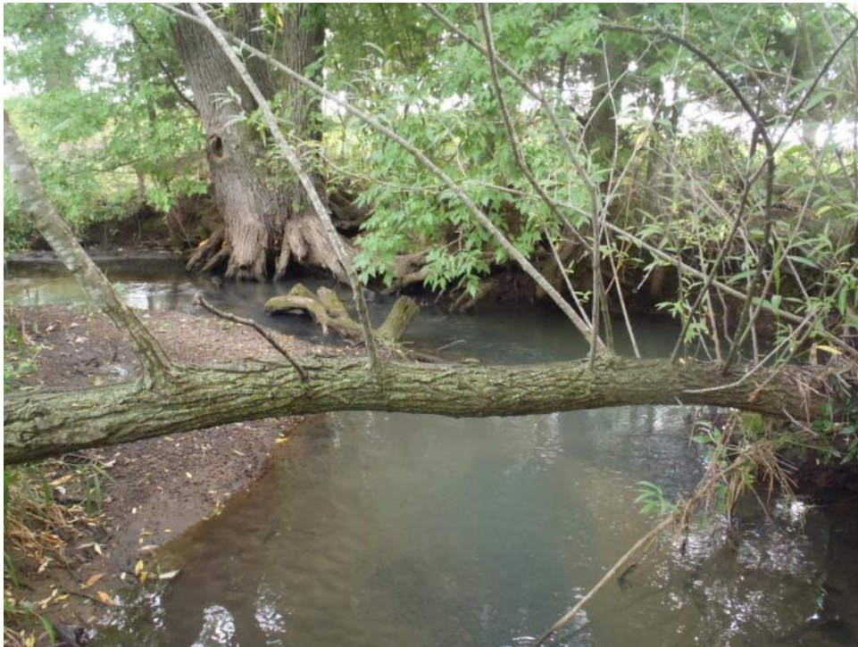
Figure 40. Eroding stream bank on the -545 reach of Threemile Creek.
