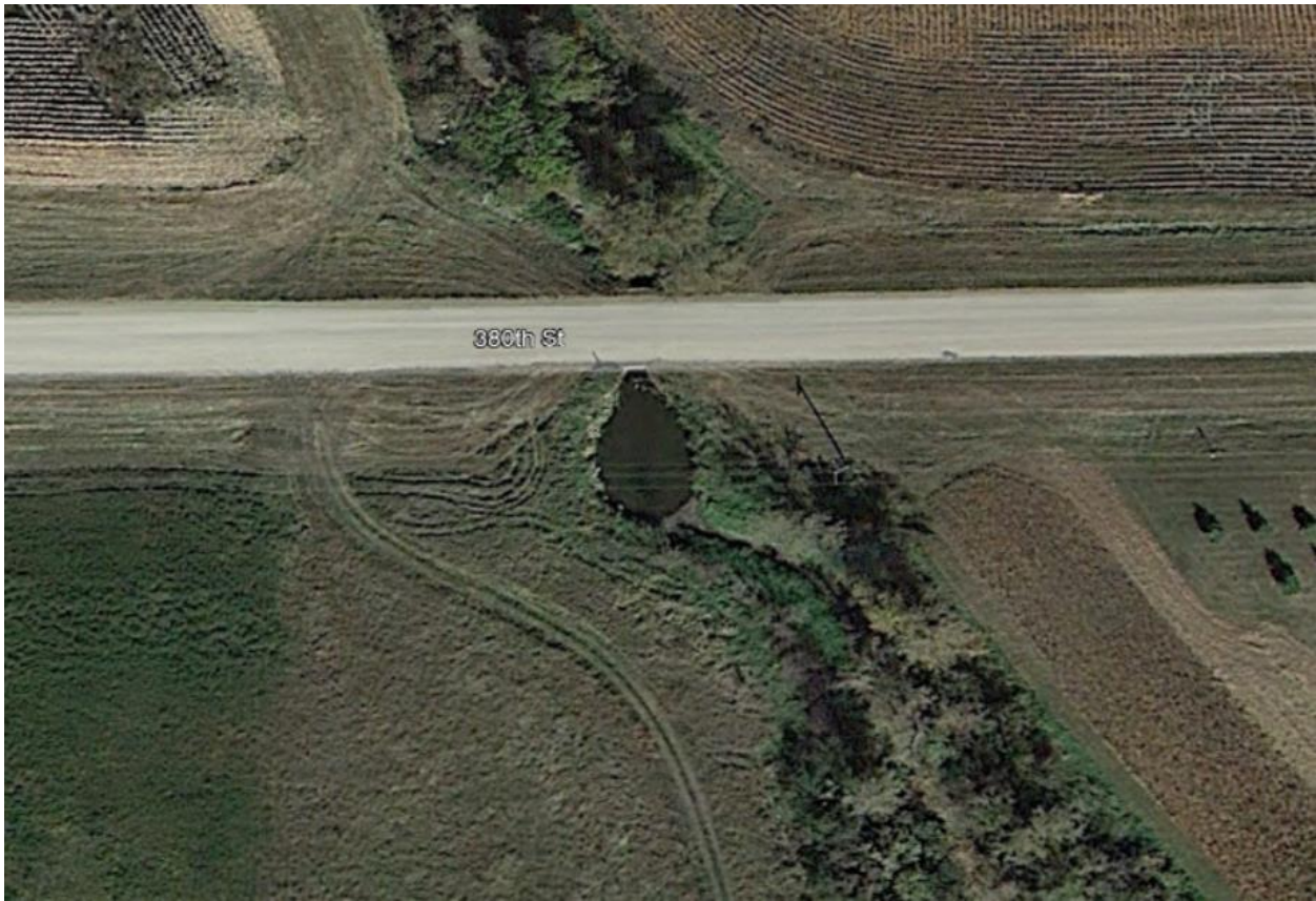
Figure 34. Plunge pool on the downstream end of the culvert crossing off 380th Street.
