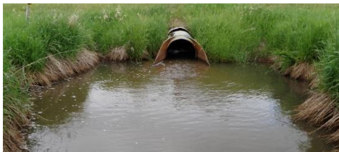
Figure 60. Culvert crossing off CR 11 in 2009.
