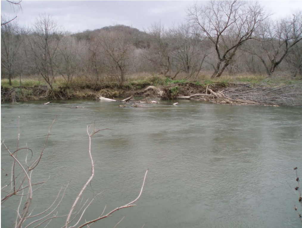
Photo 12-3. Bank erosion at Site 12.
