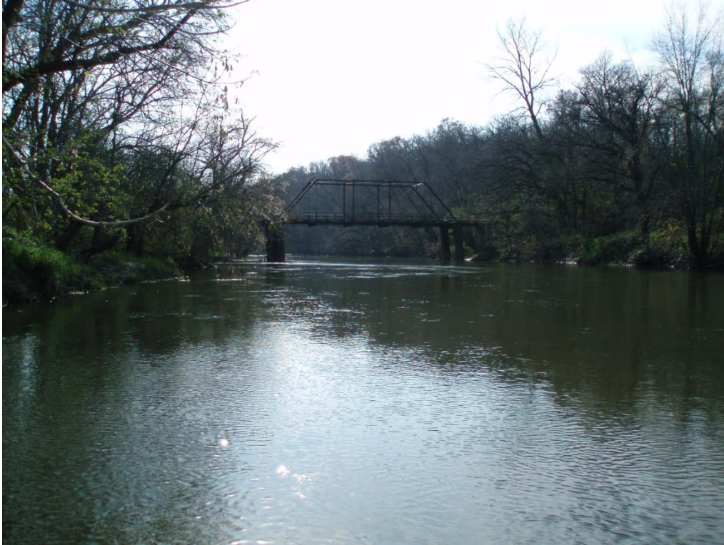
Photo 5-1. Looking upstream at Site 5.
