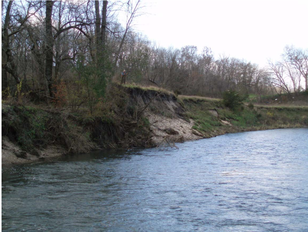
Photo 6-3. Bank erosion at Site 6.
