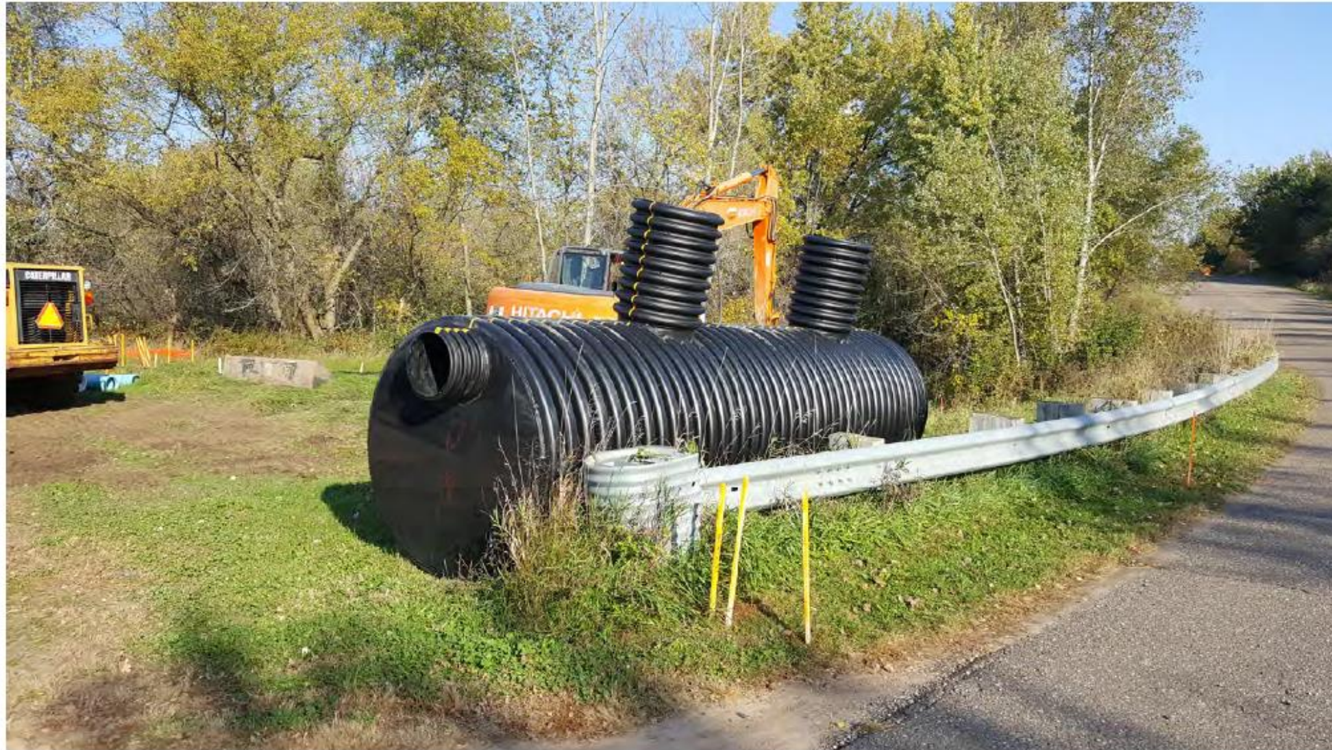
Stormwater Quality Tank Pre-Installation (EOR)
