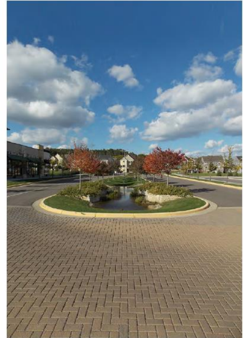
Permeable Paver Intersection in Inver Grove Heights (EOR)
