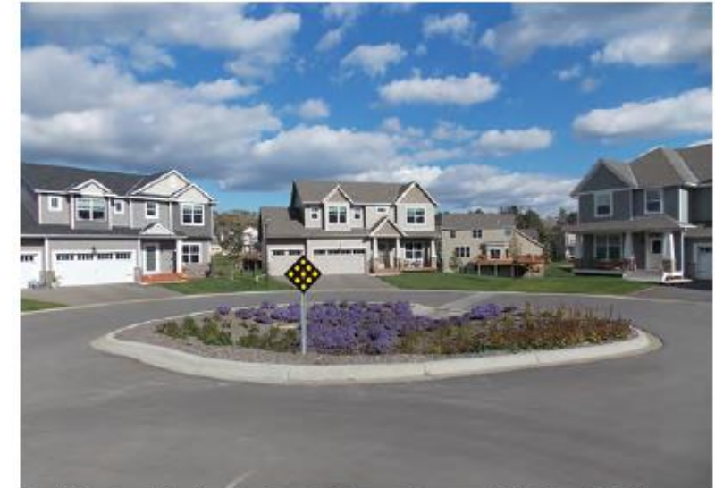
Cul-de-Sac Rain Garden in Inver Grove Heights (EOR)
