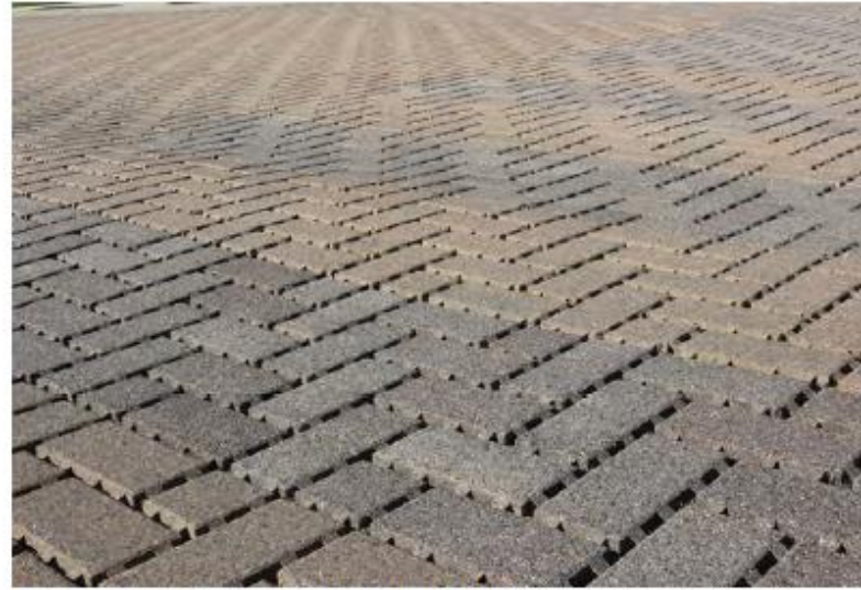
Permeable Pavers, installed (EOR)
