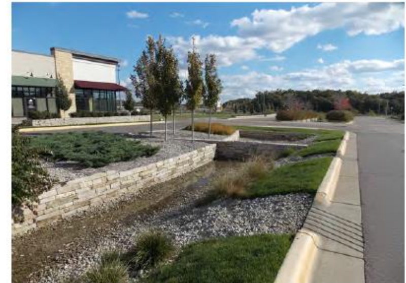
Median Rain Garden in Inver Grove Heights (EOR)
