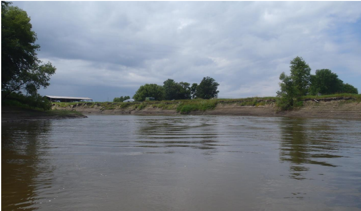
Figure 19. Example of streambank erosion in rural areas at biological monitoring station 13UM017. Photo taken by MPCA Staff August 8, 2013.
