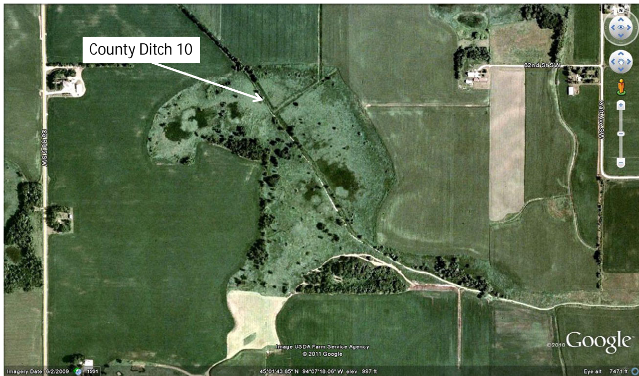
Figure 5.4. An in-line wetland that could be modified to increase water storage and improve water quality. Buffers could also be added around the perimeter.
