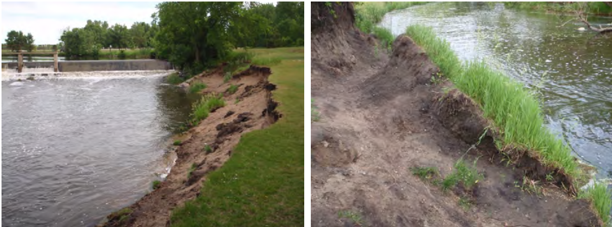
Figure 90. Photographs showing streambanks below Morris dam
