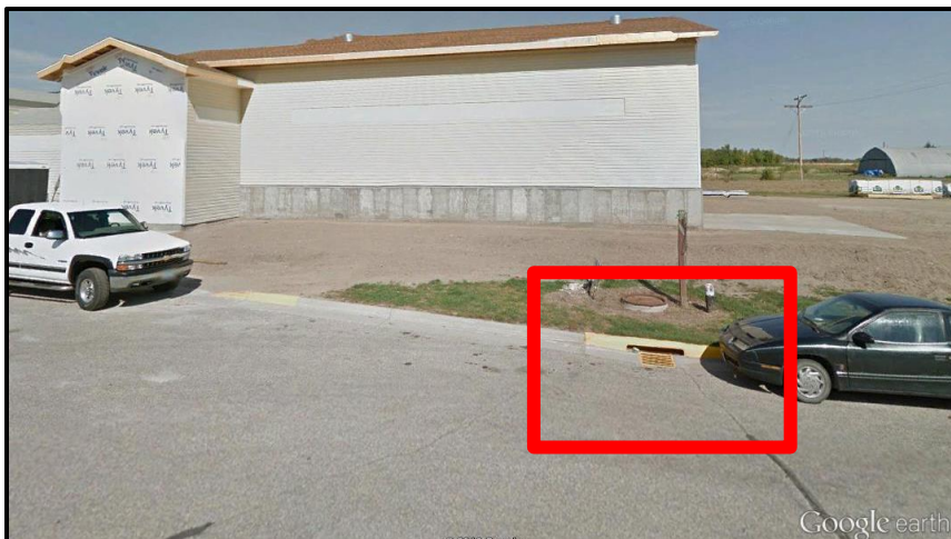
Figure 8-1. Stormwater inlet near an agricultural supply company in Grygla
