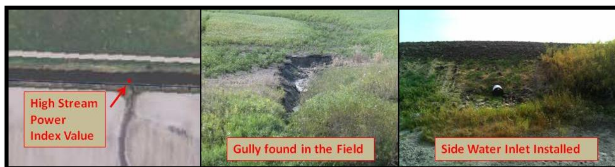
Figure 8-4. Utilization of Stream Power Index results to plan side water inlet installations
